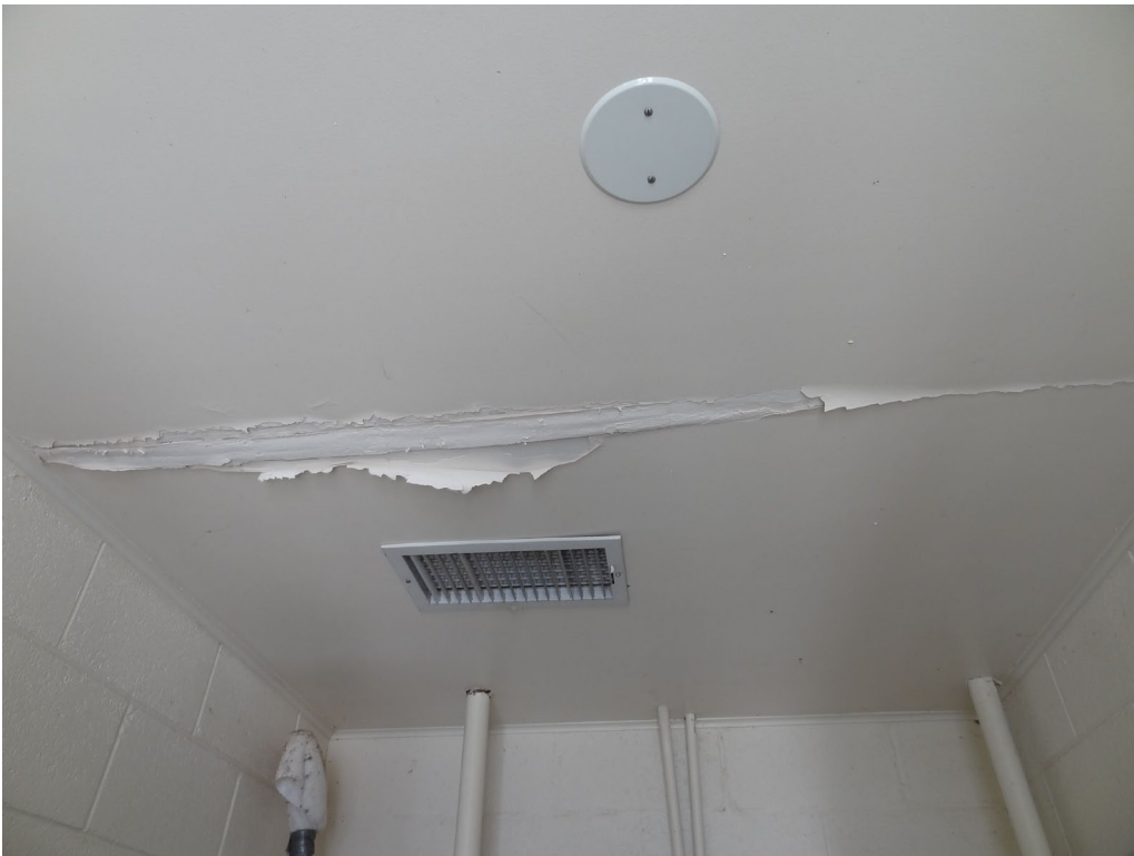
Comfort Station #1 - Building #1908 Description: Gypsum Board Repair.
