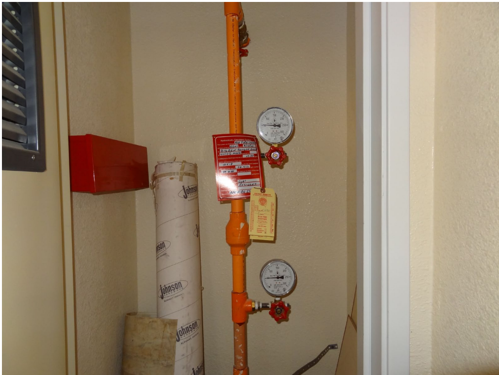
Ranger Residence #1 - Building #1907 Description: View of Fire Suppression Riser.
