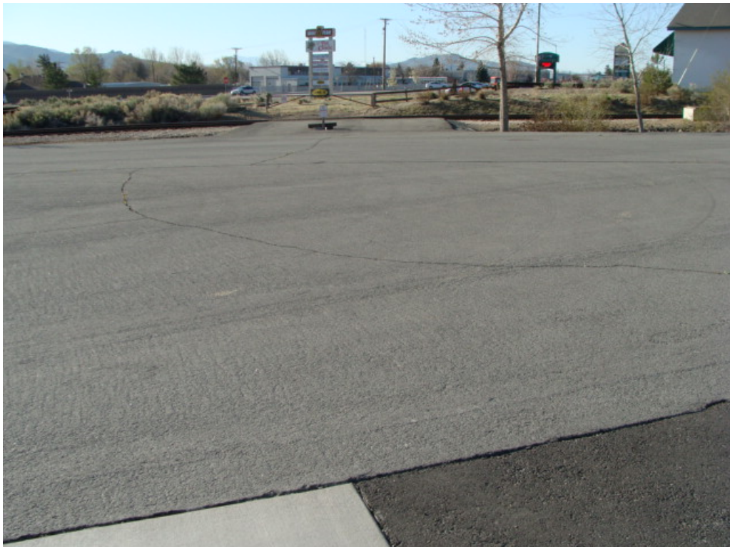
Nevada State Railroad Museum Carson City - Site #9932 Description: Crack Fill & Slurry Seal Asphalt Paving.
