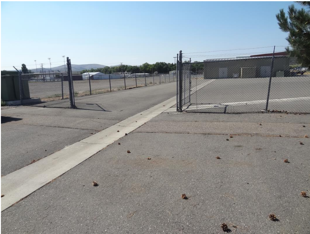
Elko Armory - Site #9937 Description: Exterior lighting needed.
