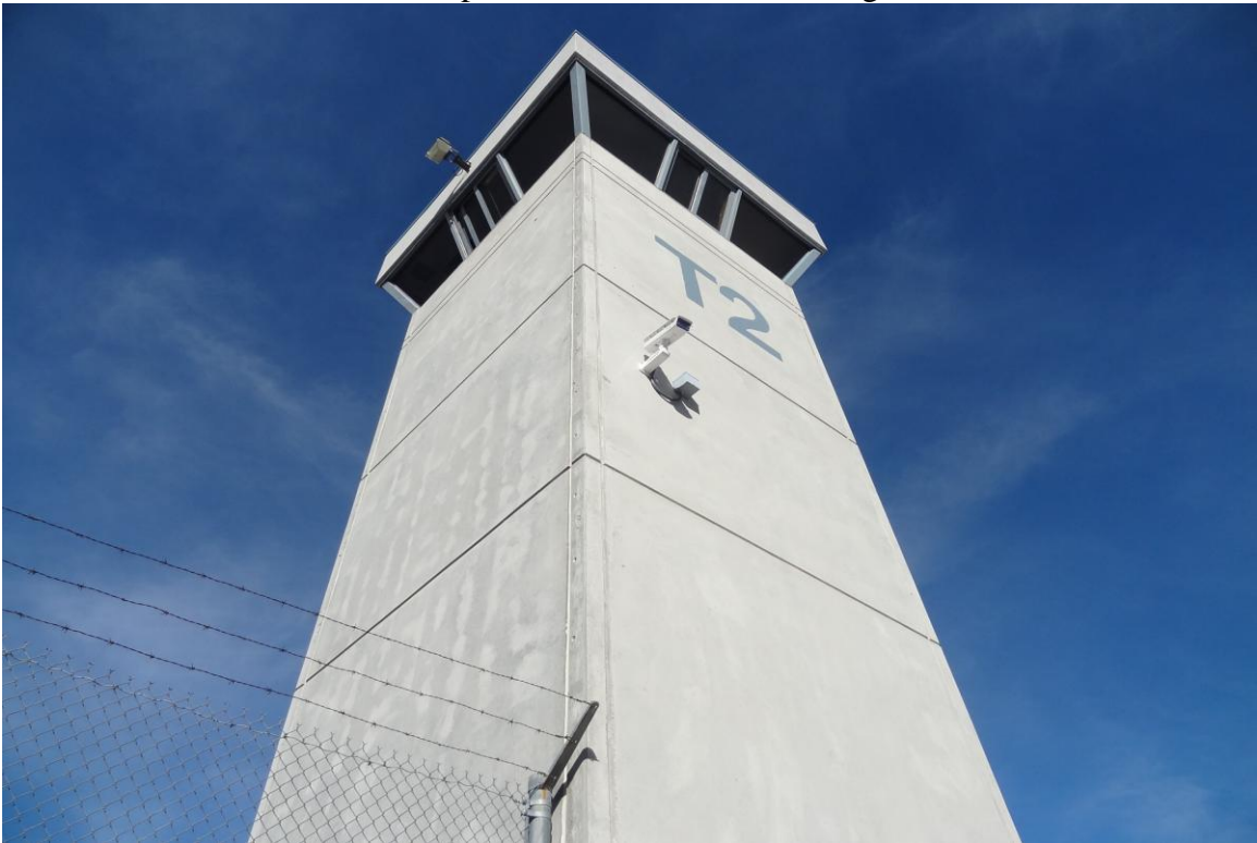
Tower 2 – FCA Building #1430 Description: Exterior of the building.
