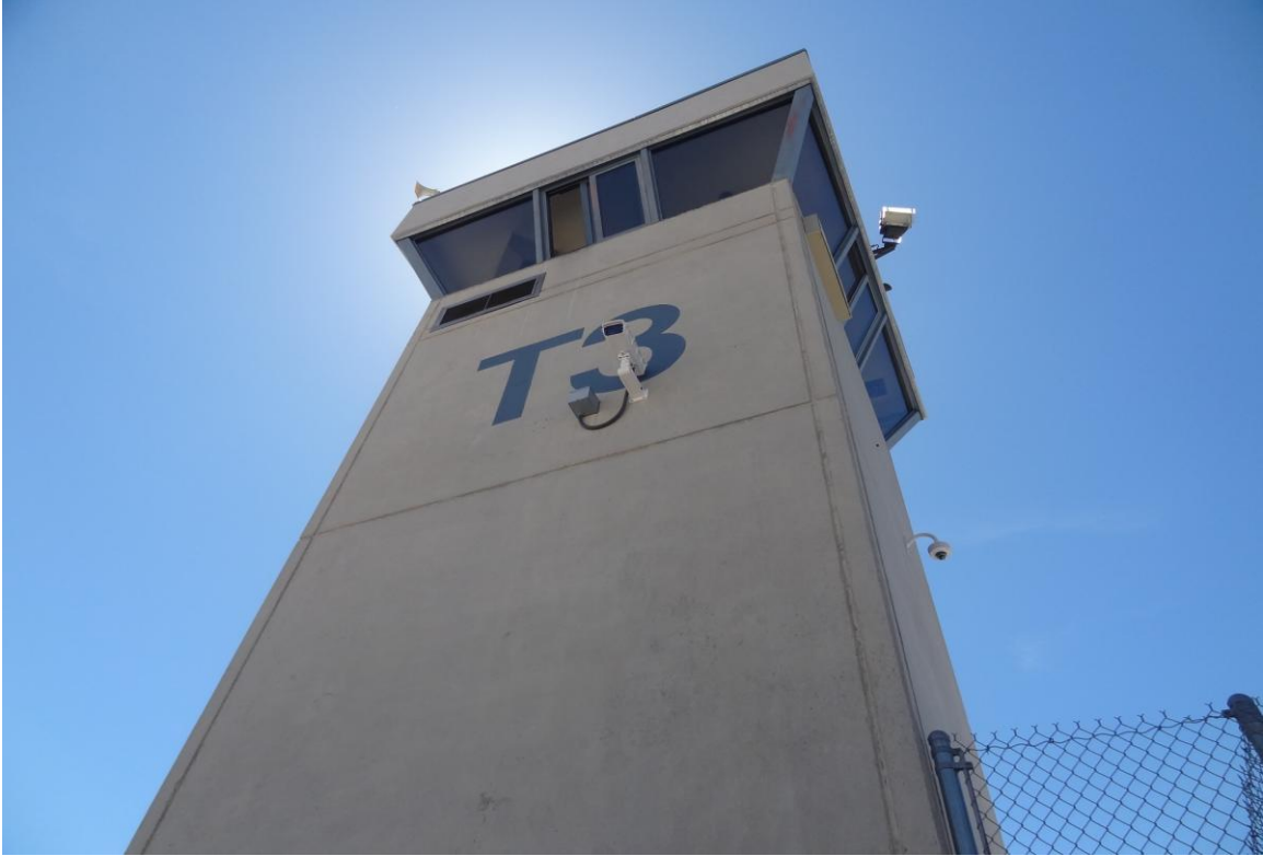
Tower 3 – FCA Building #1431 Description: Exterior of the building.
