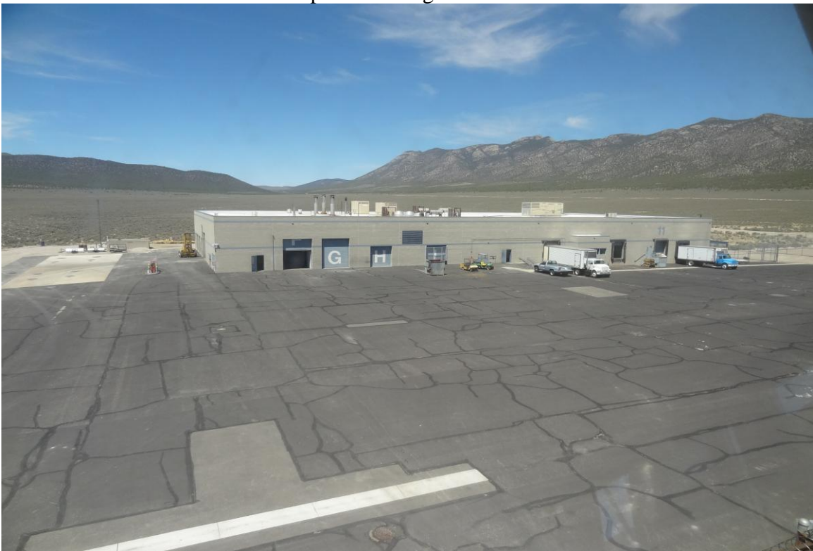
Building #11 Warehouse / Central Plant – FCA Building #1425 Description: Exterior of the building.
