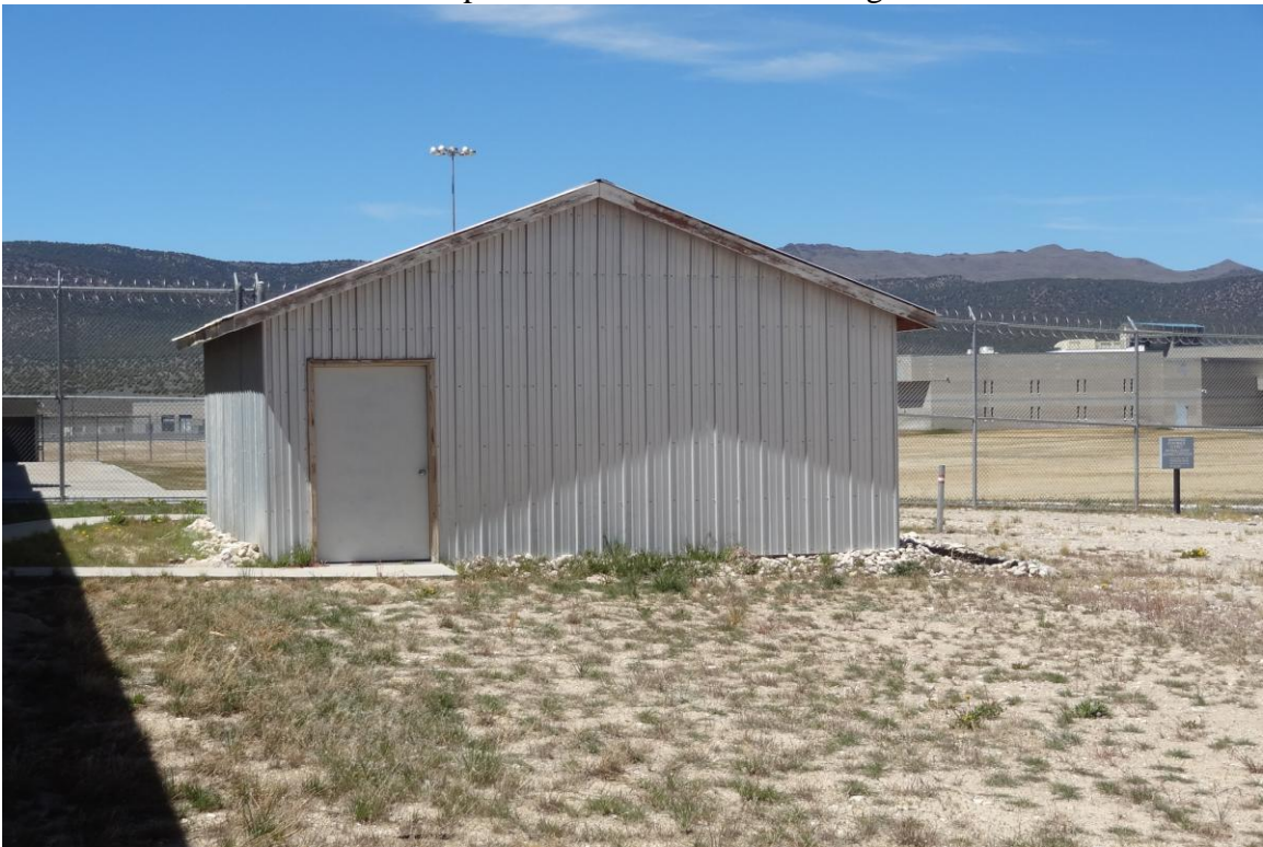
Equipment Storage – FCA Building #2242 Description: Exterior of the building.
