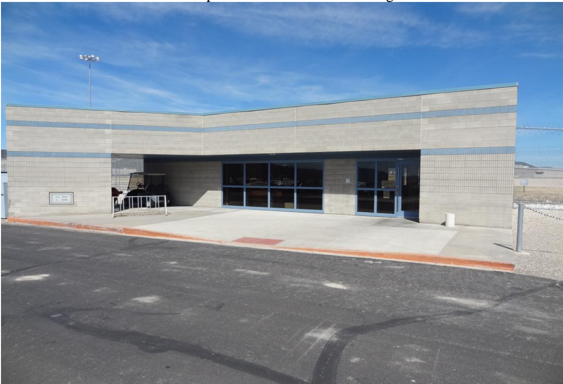
Building #14 Gatehouse – FCA Building #1428 Description: Exterior of the building.
