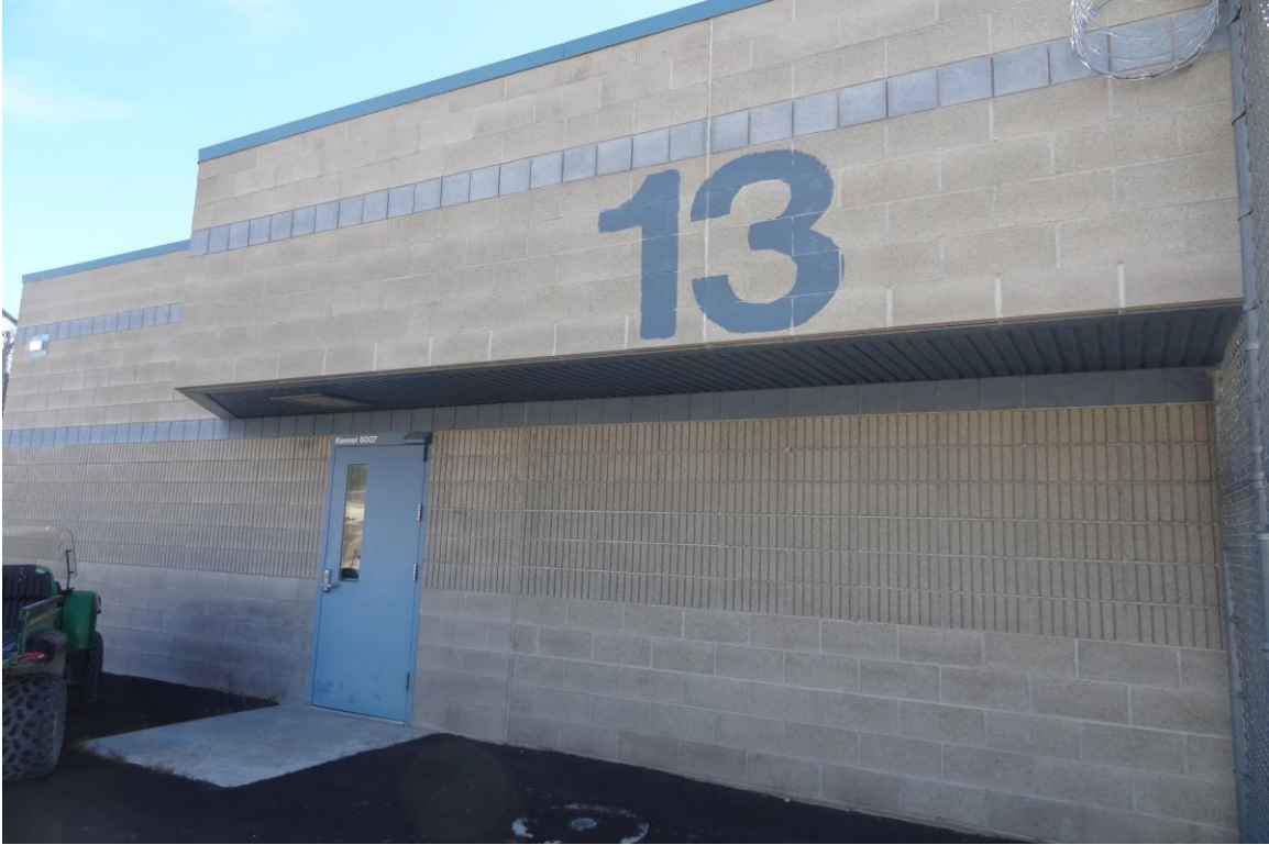
Building #13 Armory – FCA Building #1427 Description: Exterior of the building.
