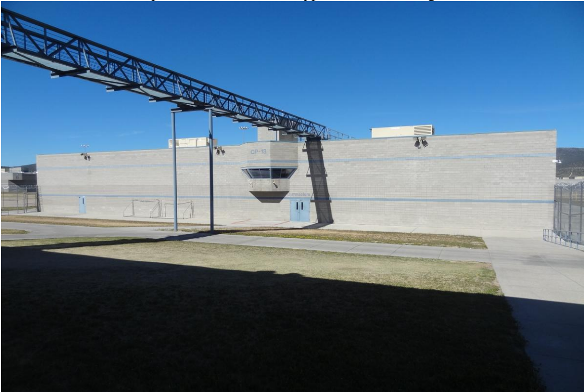
Building #9 Scheduled Services – FCA Building #1423 Description: Exterior of the building.
