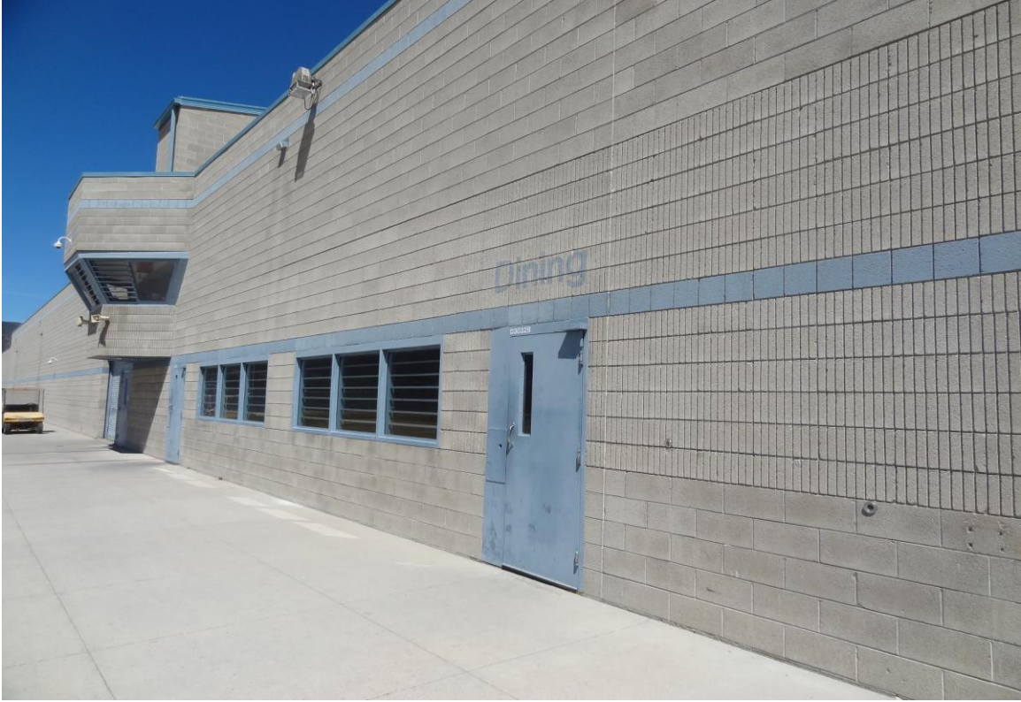
Building #10 Work & Recreation – FCA Building #1424 Description: Exterior of the building.
