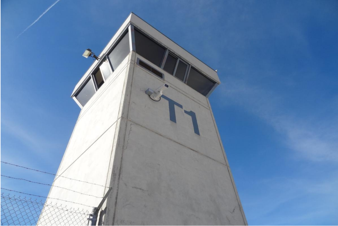
Tower 1 – FCA Building #1429 Description: Exterior of the building.
