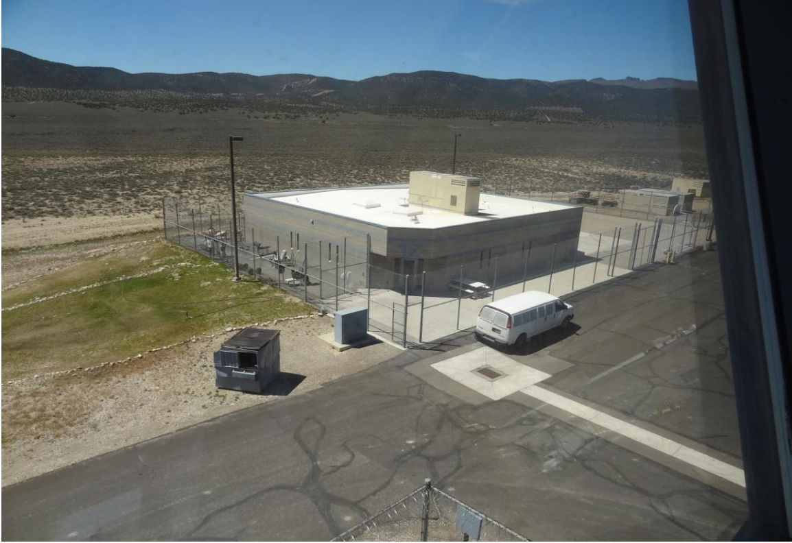
Building #12 Trustee Dormitory – FCA Building #1426 Description: Exterior of the building.
