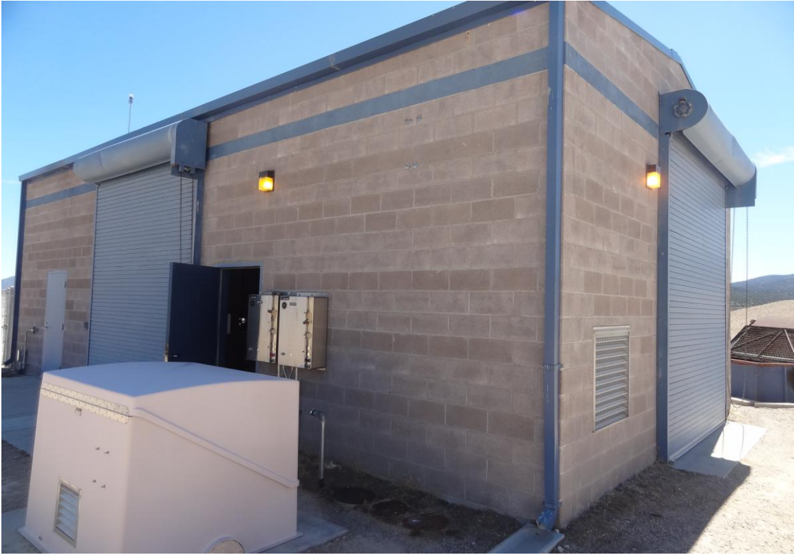
ESP Sewage Grinder Building – FCA Building #1617 Description: Exterior of the building.
