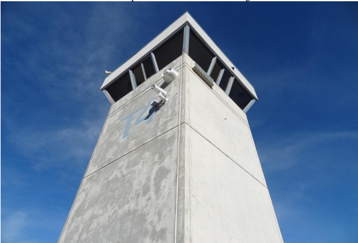
Tower 4 – FCA Building #1432 Description: Exterior of the building.
