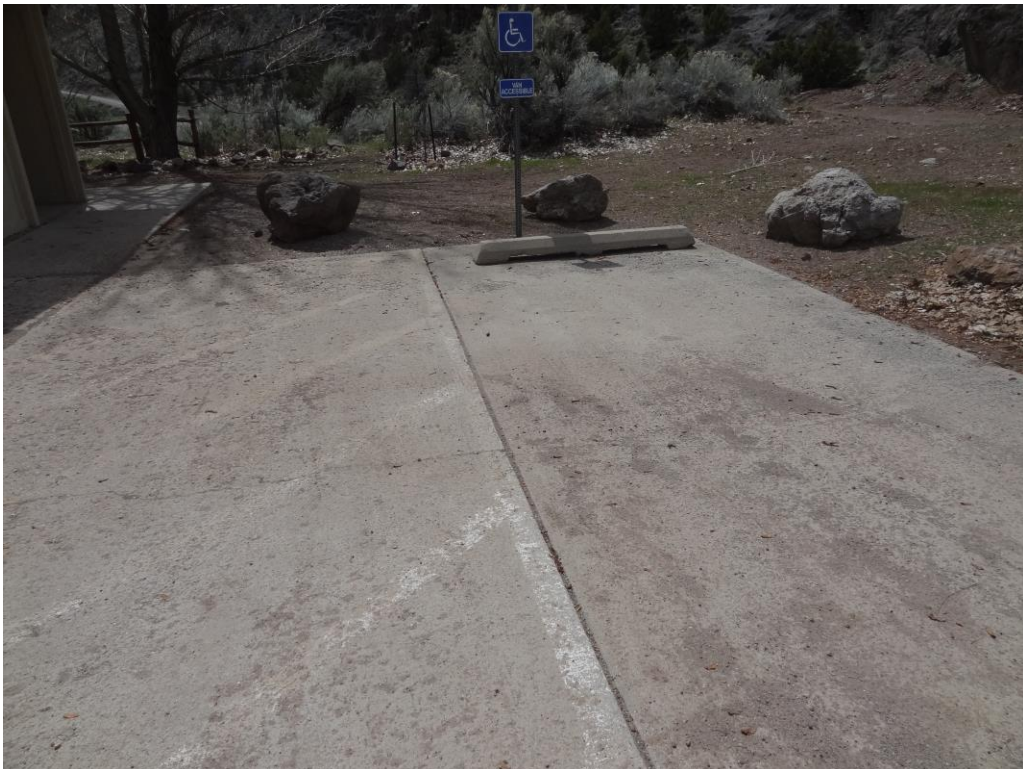
Comfort Station #1 - Building #1177 Description: Deteriorated and non-compliant ADA Parking Space.
