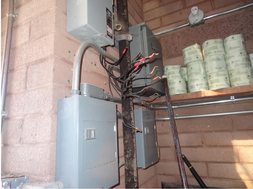
Comfort Station #3 - Building #0509 Description: Wiring cleanup needed.
