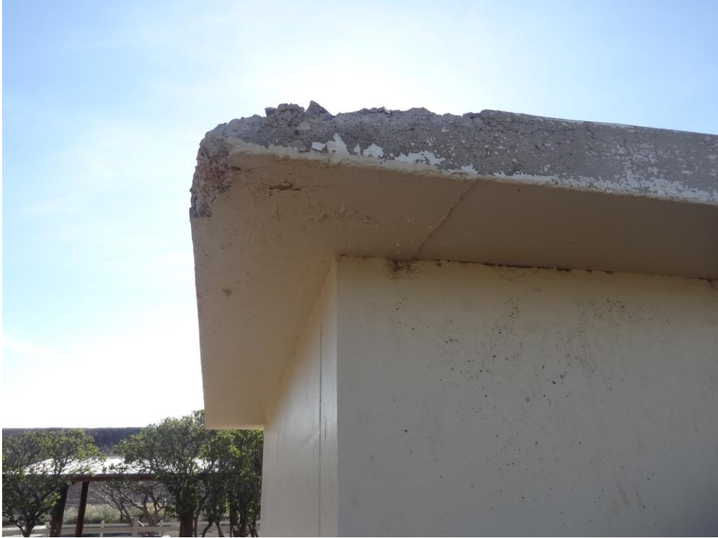
Park Well House - Building #1065 Description: Concrete patch/ roofing needed.
