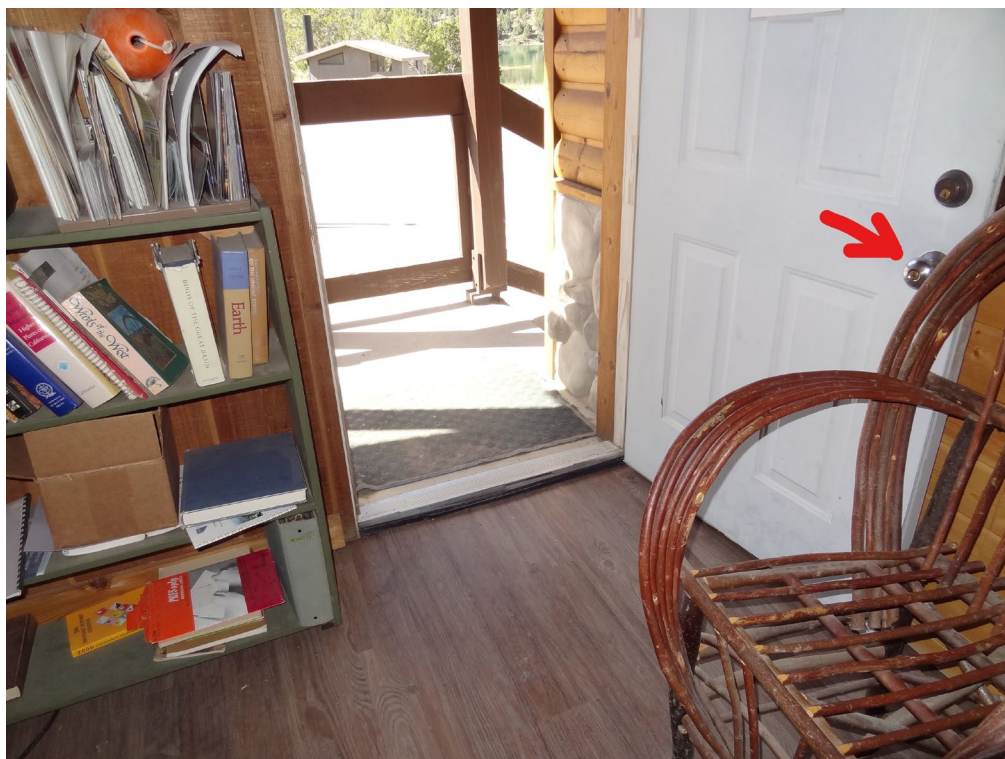
Cave Lake Office / Shop - Building #1284 Description: ADA Upgrades, Lever Handles Needed.
