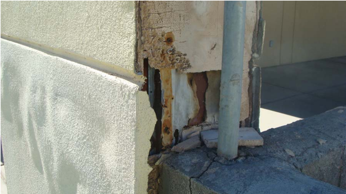
CYC School - New - Building #2001 Description: Water damaged EIFS.
