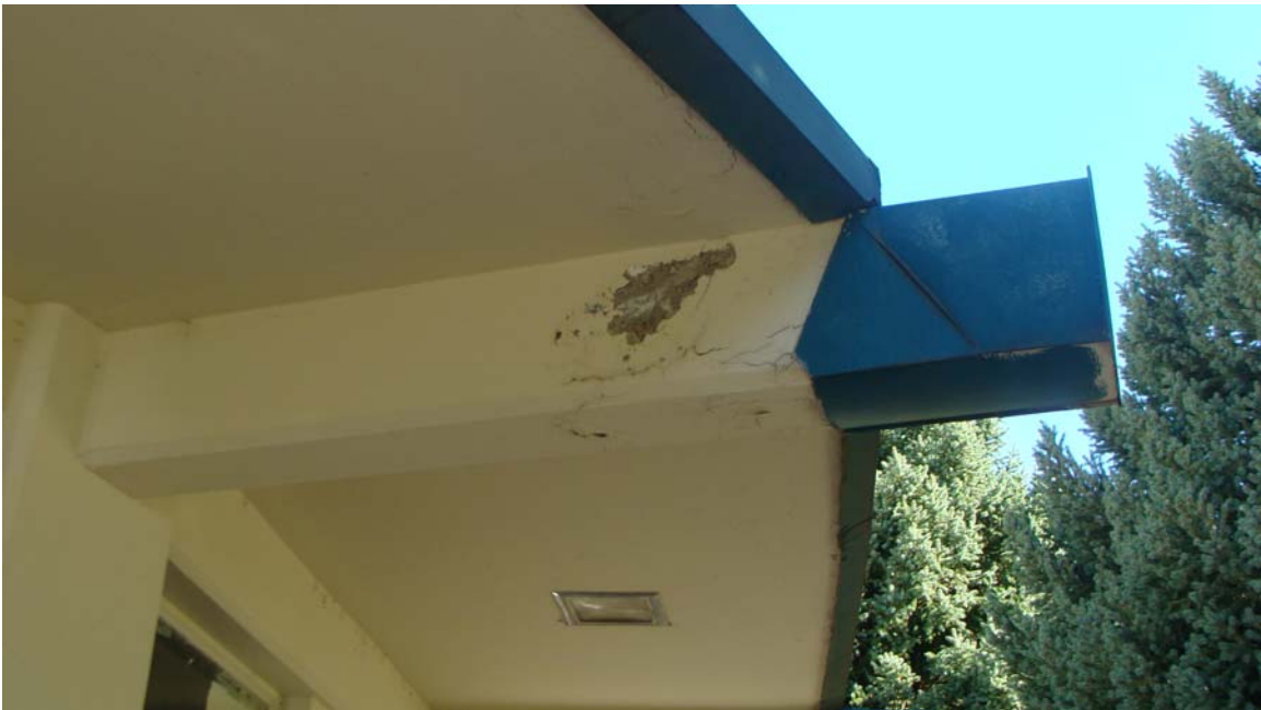
CYC Beowawe Dormitory - Building #0212 Description: Damaged concrete roof support.
