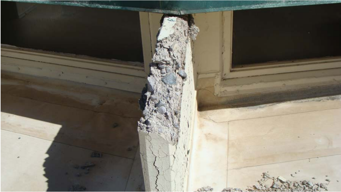
CYC Aurora Dormitory - Building #0211 Description: Damaged concrete roof support.
