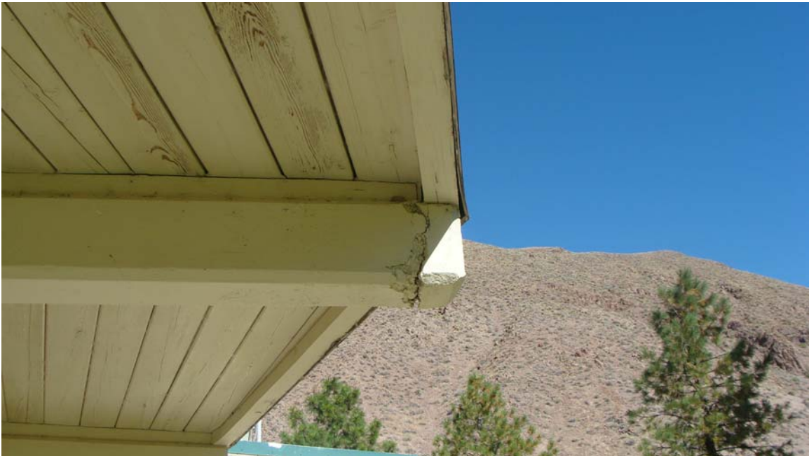
CYC Lincoln Dormitory - Building #0217 Description: Damaged concrete roof support.
