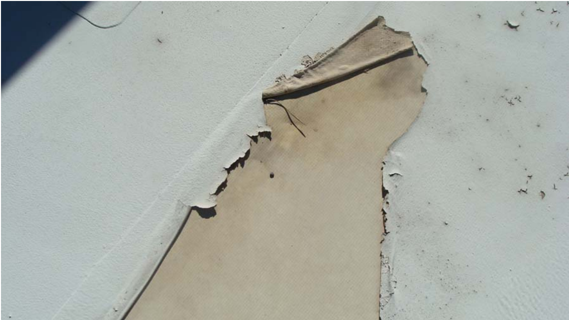
CYC Culinary / Dining / Gym / Laundry - Building #0221 Description: Damaged roof membrane.
