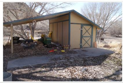
The CYC Industrial Arts Storage is a wood framed structure with an asphalt composition roofing system on a concrete slab-ongrade foundation.
