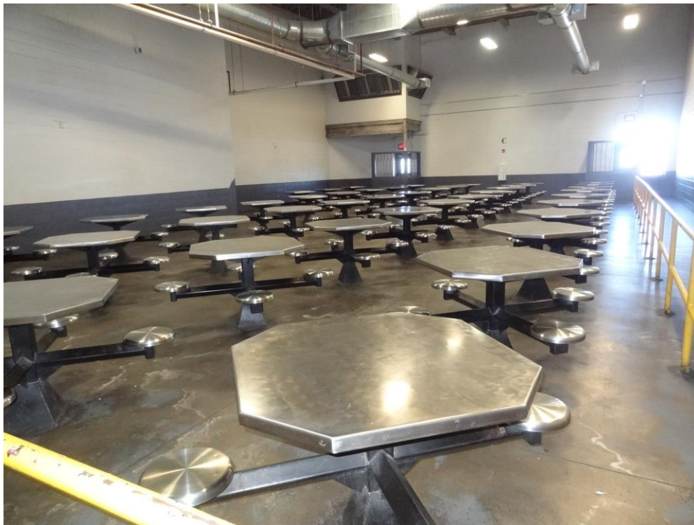
Inmate Services/ Culinary/ Dining - Building #2091 Description: ADA table upgrade needed.
