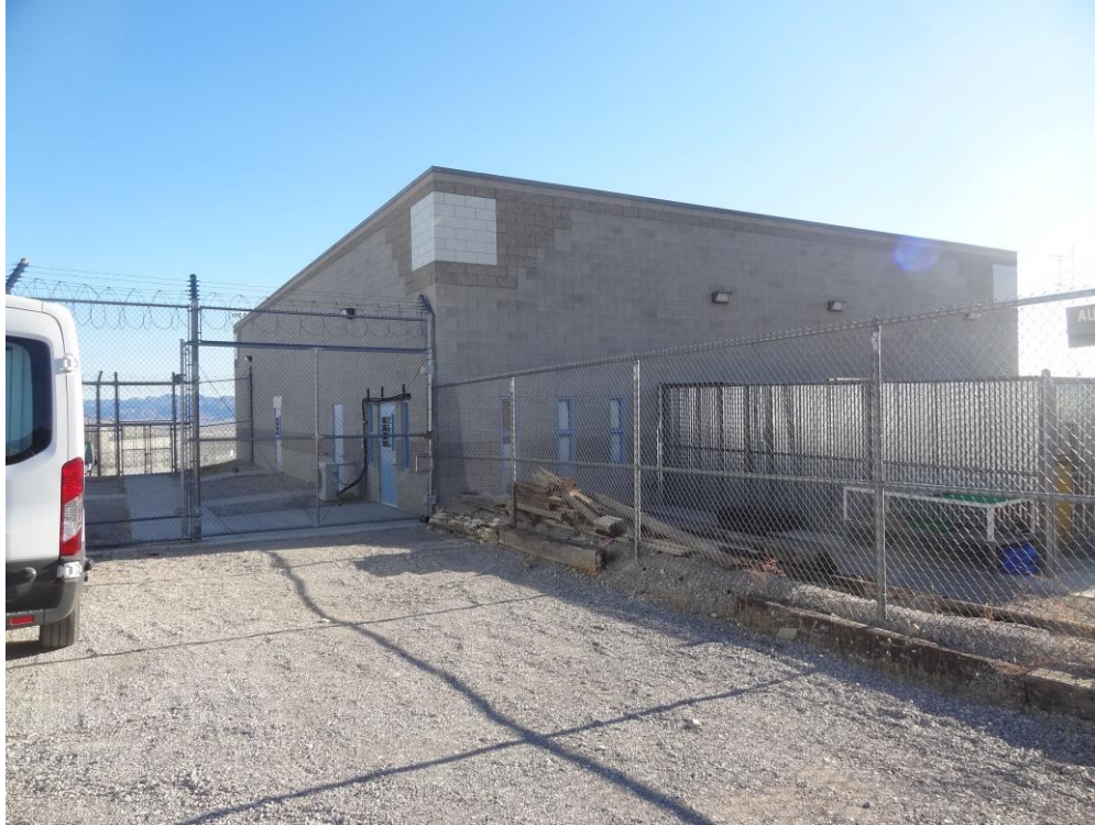
Armory/ Emergency Response - Building #2098 Description: Exterior finishes.
