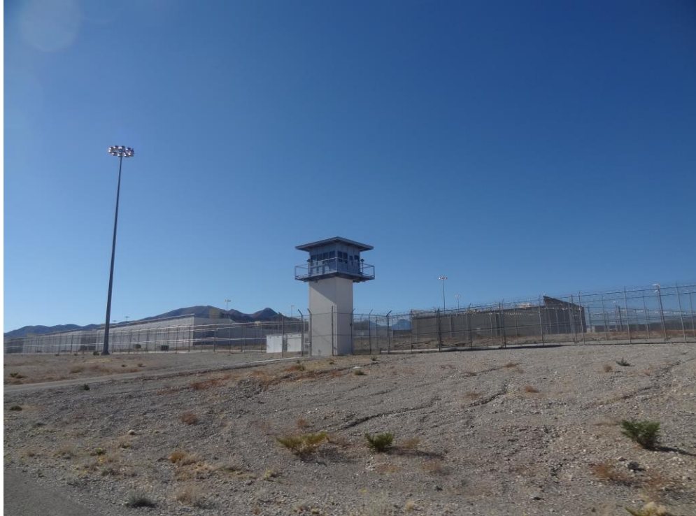
Tower #4 - Building #2177 Description: Exterior finishes.
