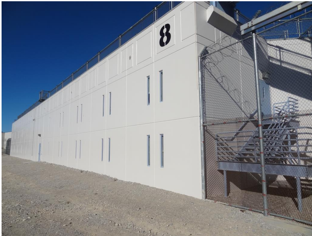
Housing Unit #8 - Building #2172 Description: Exterior finishes.
