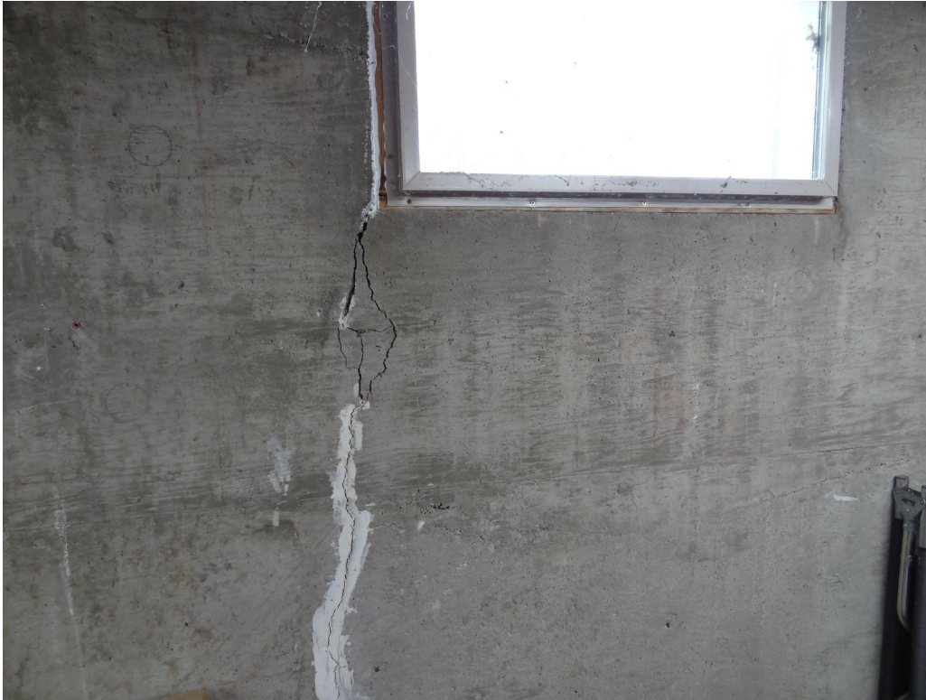
Supervisor's Residence - Building #0903 Description: Basement Concrete Repairs.
