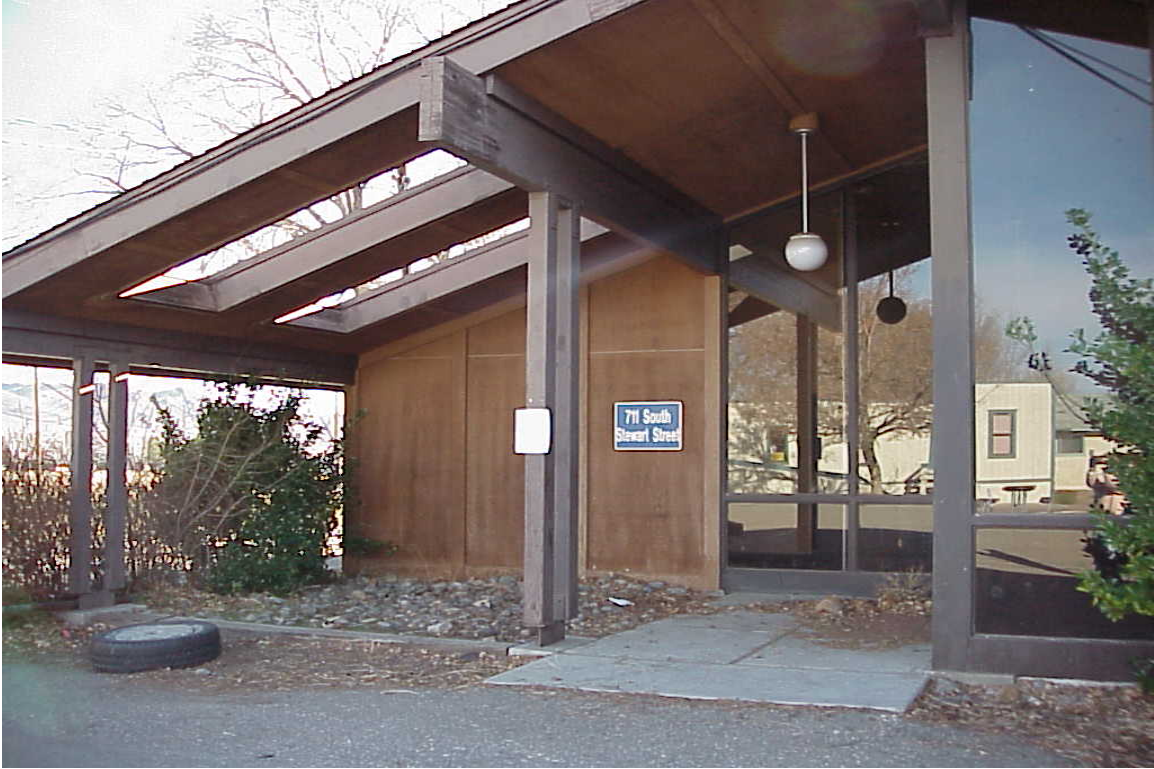
Child & Family Services Division/Rehabilitation Building (Vacant) - Building #0297 Description: The exterior of the building.
