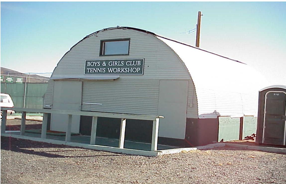
Child & Family Services Division/Quonset - Building #2313 Description: The exterior of the building.
