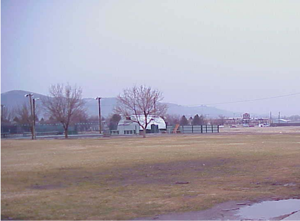
Child & Family Services Division/Quonset - Building #2313 Description: The exterior of the building.
