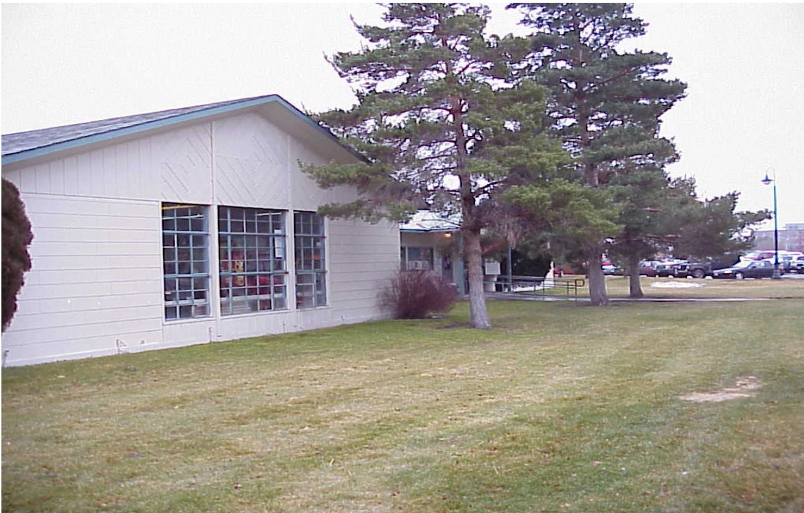
Child & Family Services Division/Boys & Girls Club - Building #0294 Description: The exterior of the building.
