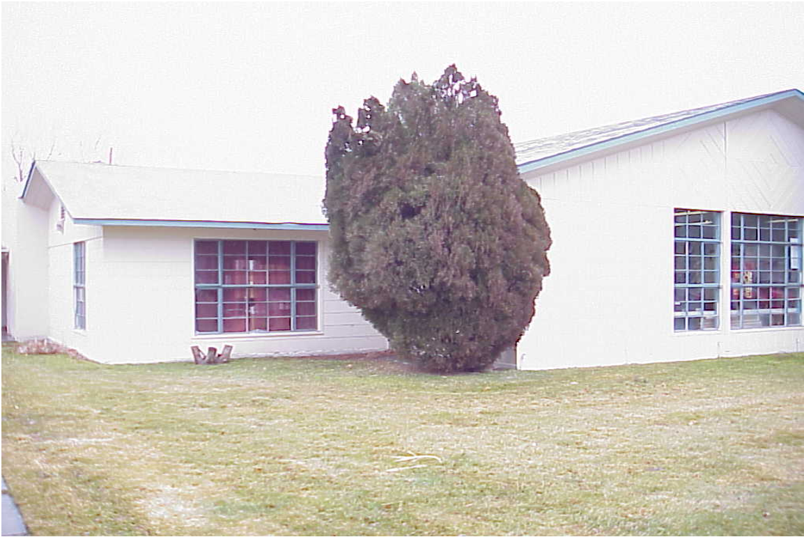
Child & Family Services Division/Boys & Girls Club - Building #0294 Description: The exterior of the building.
