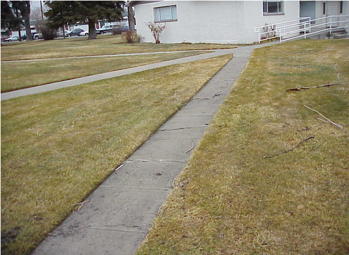
Child & Family Services Division Site #9955 Description: Typical sidewalk at site.
