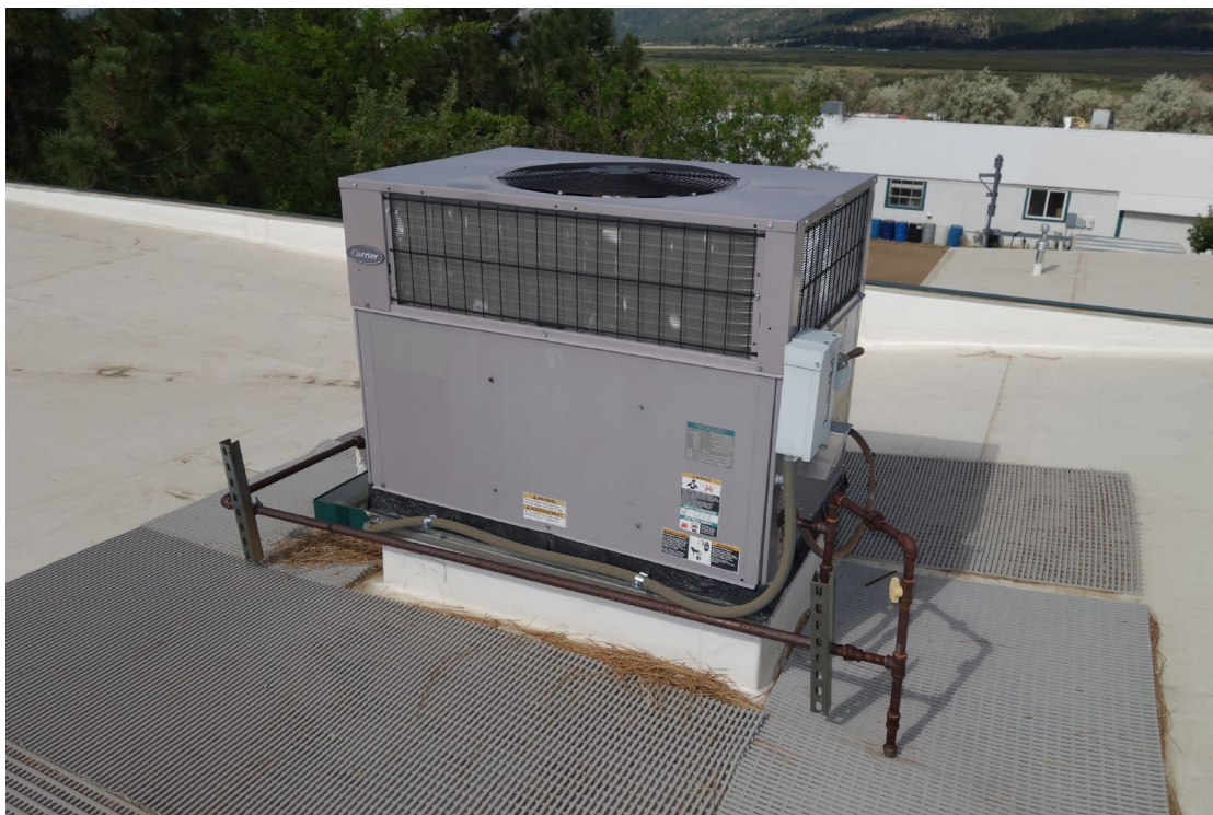
Western Area Headquarters – FCA Building #1655 Description: HVAC Rooftop Unit Replacement Planning Needed.
