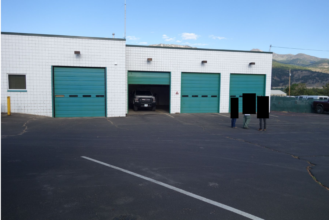
Western Area Headquarters – FCA Building #1655 Description: Bollard Protection at Overhead Doors Needed.
