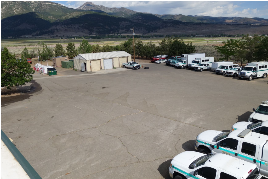
NDF Western Area Headquarters Site – FCA Site #9957 Description: Crack Fill & Seal Parking Areas Needed.
