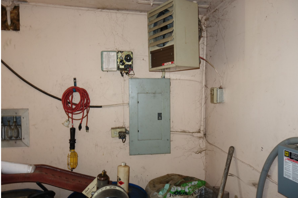
HQ Garden Equipment Storage – FCA Building #2348 Description: Improper Non-Metallic Sheathed Electrical Cable.
