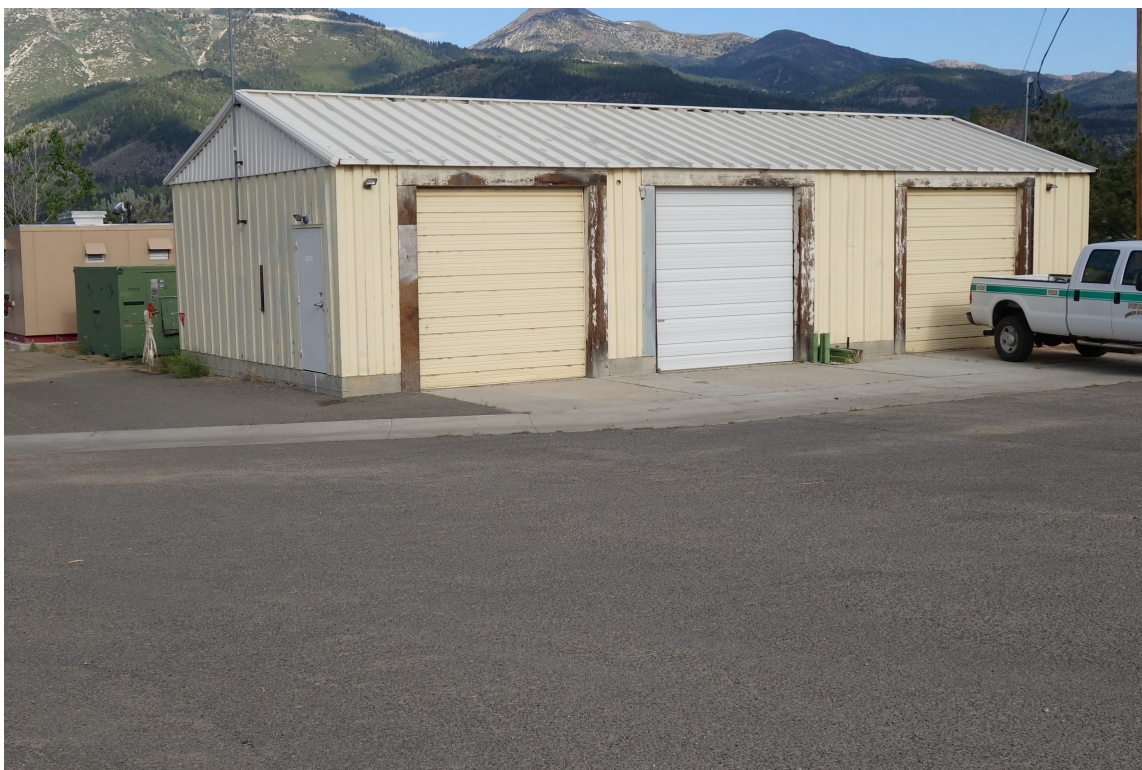
HQ Welding Shop – FCA Building #2339 Description: Exterior of Building and Missing Door Landing.
