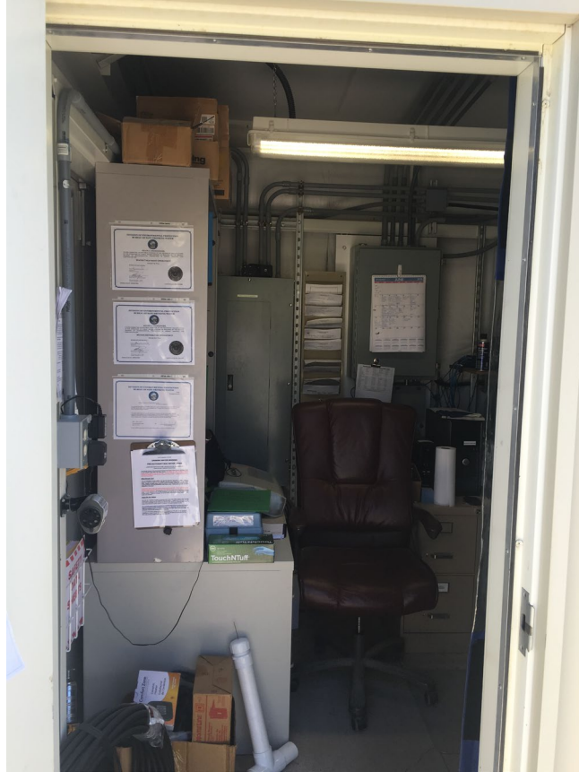
Water Treatment Plant- Building #3054 Description: Arc Flash & Breaker Coordination Study Needed.
