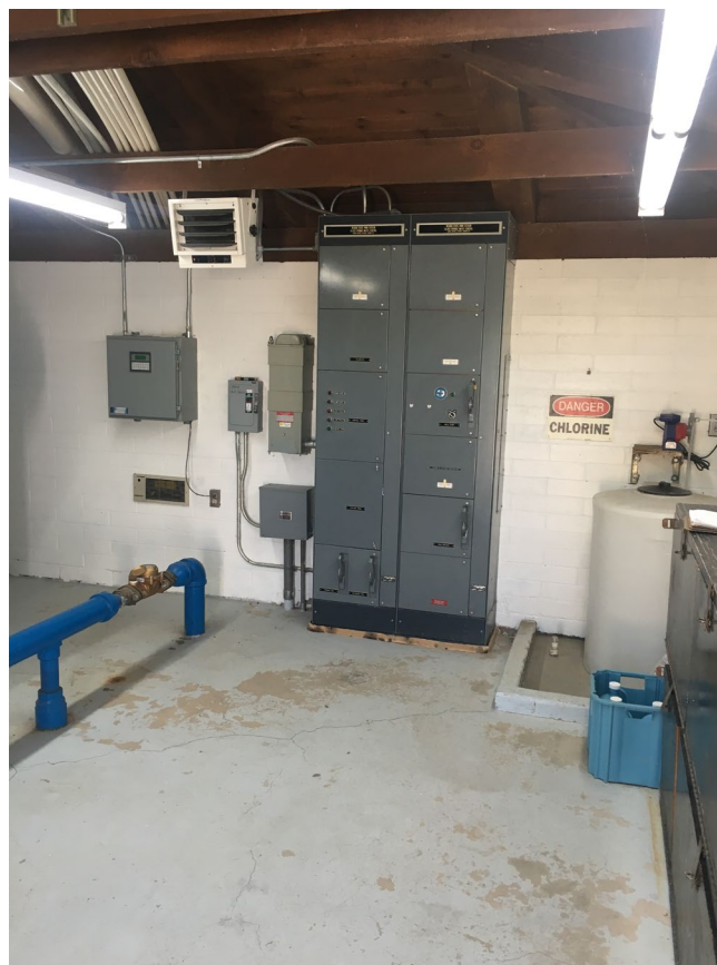
SS Mechanical Building North - Building #1347 Description: Arc Flash & Breaker Coordination Study Needed.
