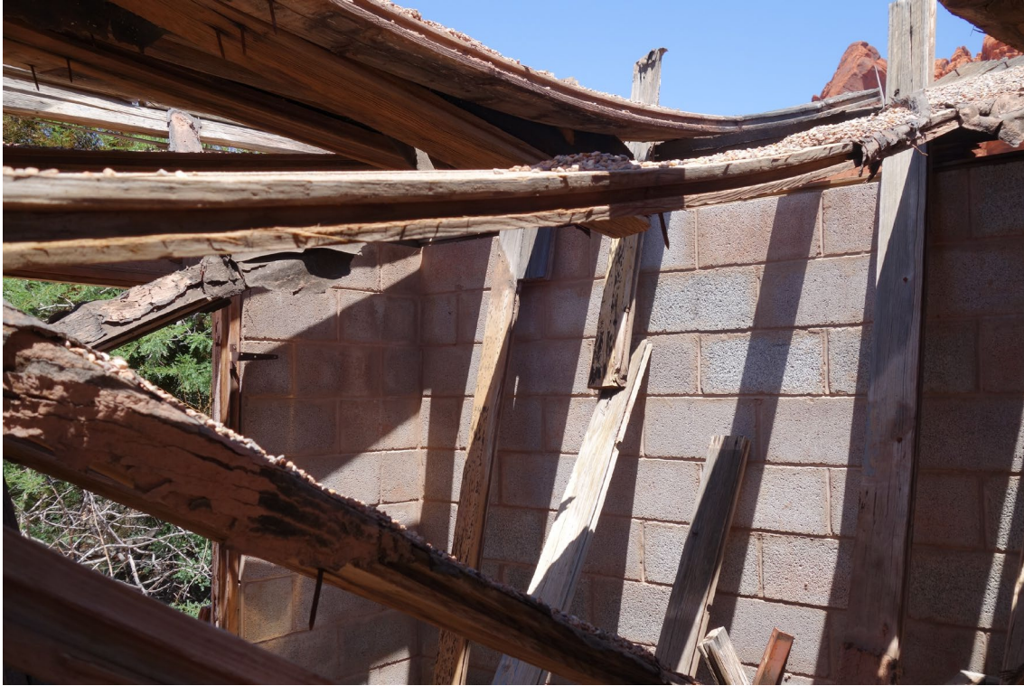
VOF Storage #2 – FCA Building #0557 Description: Interior of the Building – Recommend Demolishing.
