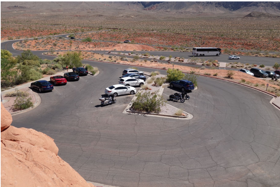
Valley of Fire State Park – FCA Site #9963 Description: Crack Fill & Slurry Seal Asphalt Paving Areas Sitewide.
