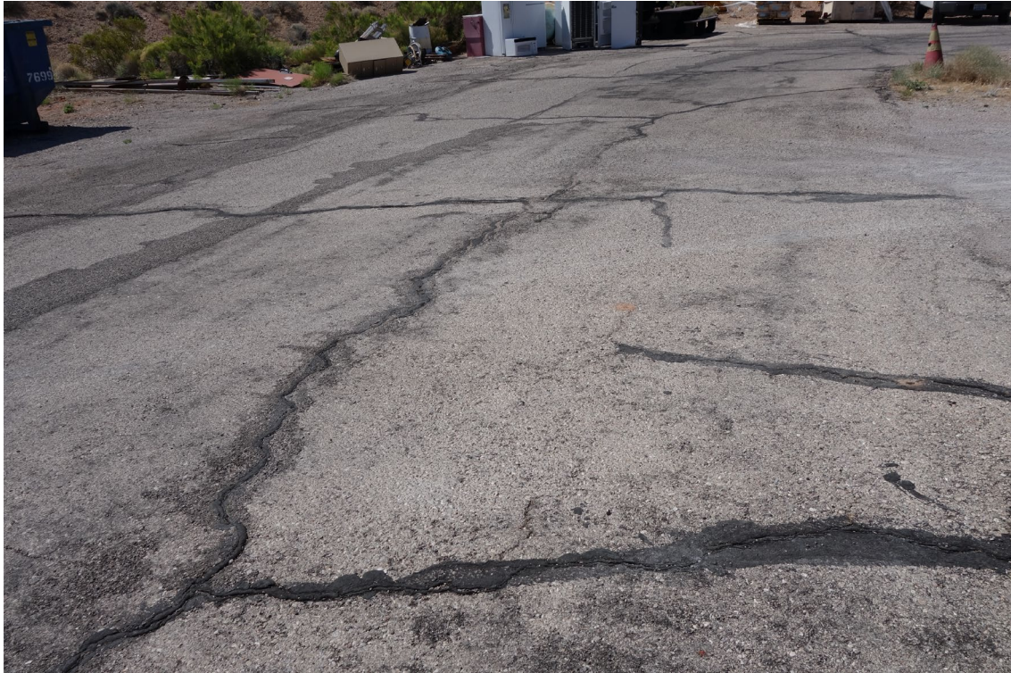
Valley of Fire State Park – FCA Site #9963 Description: Maintenance Area Pavement Replacement Needed.
