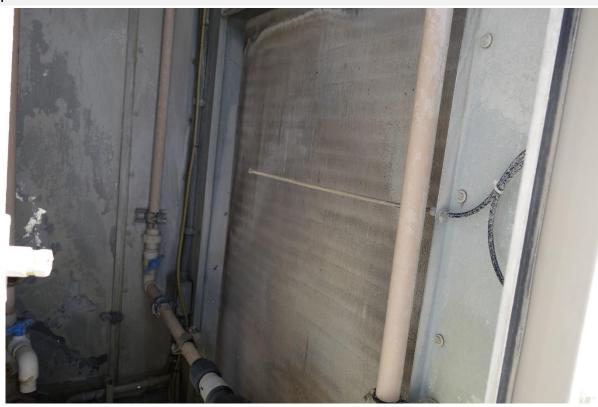
showing signs of corrosion likely caused by the same moisture carry-over. This project will fund the removal and replacement of the heating coils, a full AHU maintenance rehabilitation, new blow-down controls on the evaporative sump, water treatment (Nu-Calgon slow dissolving scale and corrosion inhibitor) and air balance. With proper maintenance, this project should restore the AHU to its expected useful life.
