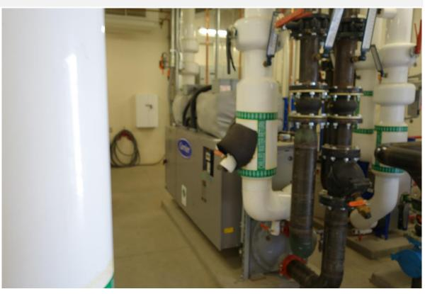
existing central plant equipment including chiller, cooling tower, chilled water heat exchanger, boilers, water heaters and associated pumps and accessories.
