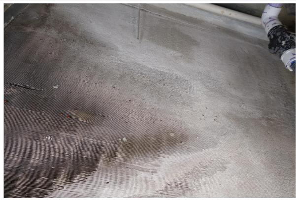
showing signs of corrosion likely caused by the same moisture carry-over. This project will fund the removal and replacement of the heating coil, a full AHU maintenance rehabilitation, new blow-down controls on the evaporative sump, water treatment (Nu-Calgon slow dissolving scale and corrosion inhibitor) and air balance. With proper maintenance, this project should restore the AHU to its expected useful life.
