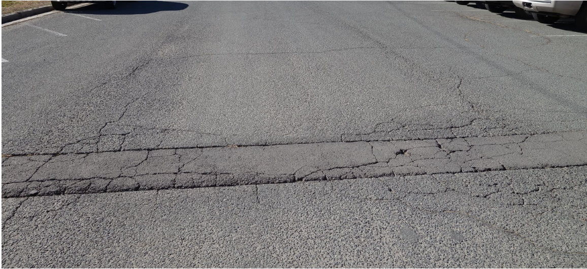
Stewart Campus Site – FCA Site #9971 Description: Crack fill and seal site wide.
