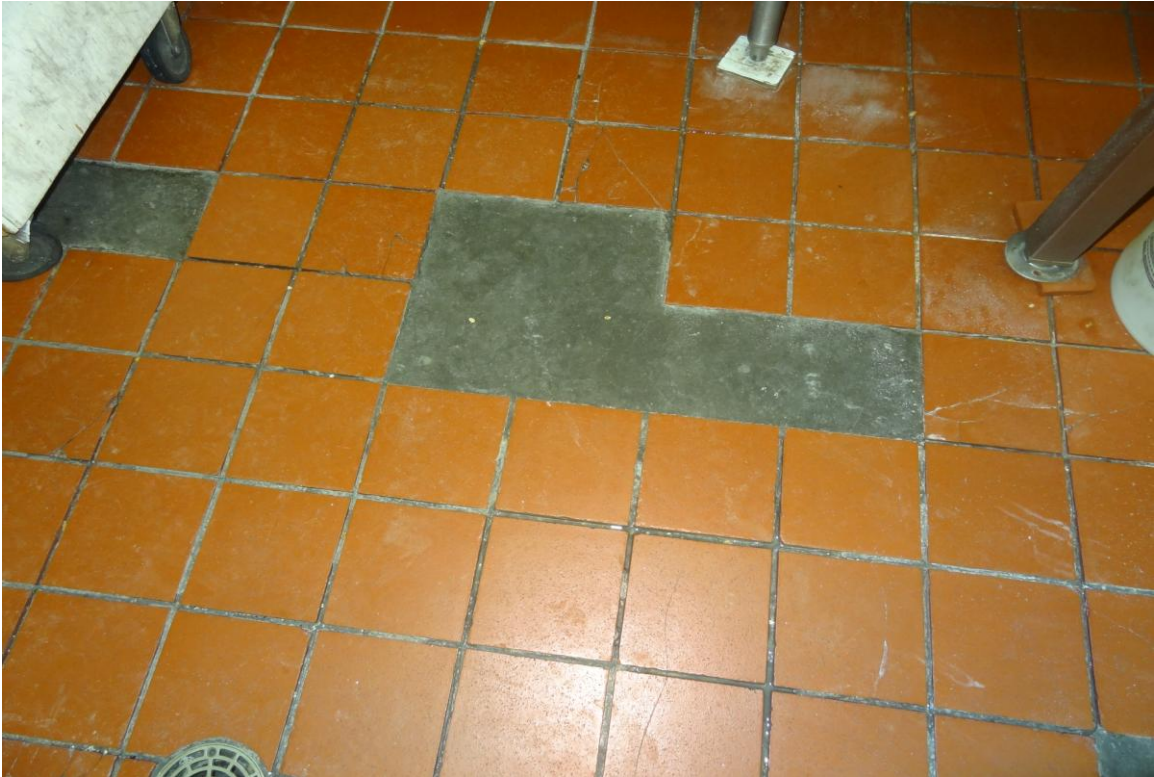
Carlin Conservation Camp Housing Unit – FCA Building #0697 Description: Missing culinary floor tiles.
