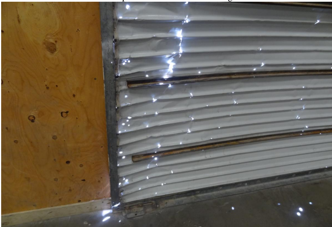
CCC Multi-Purpose Building – FCA Building #1580 Description: Over head coiling door in need of replacement.
