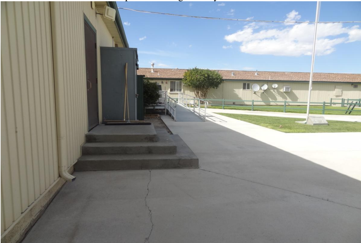
Carlin Conservation Camp Housing Unit – FCA Building #0697 Description: Exterior stairs in need of handrails.
