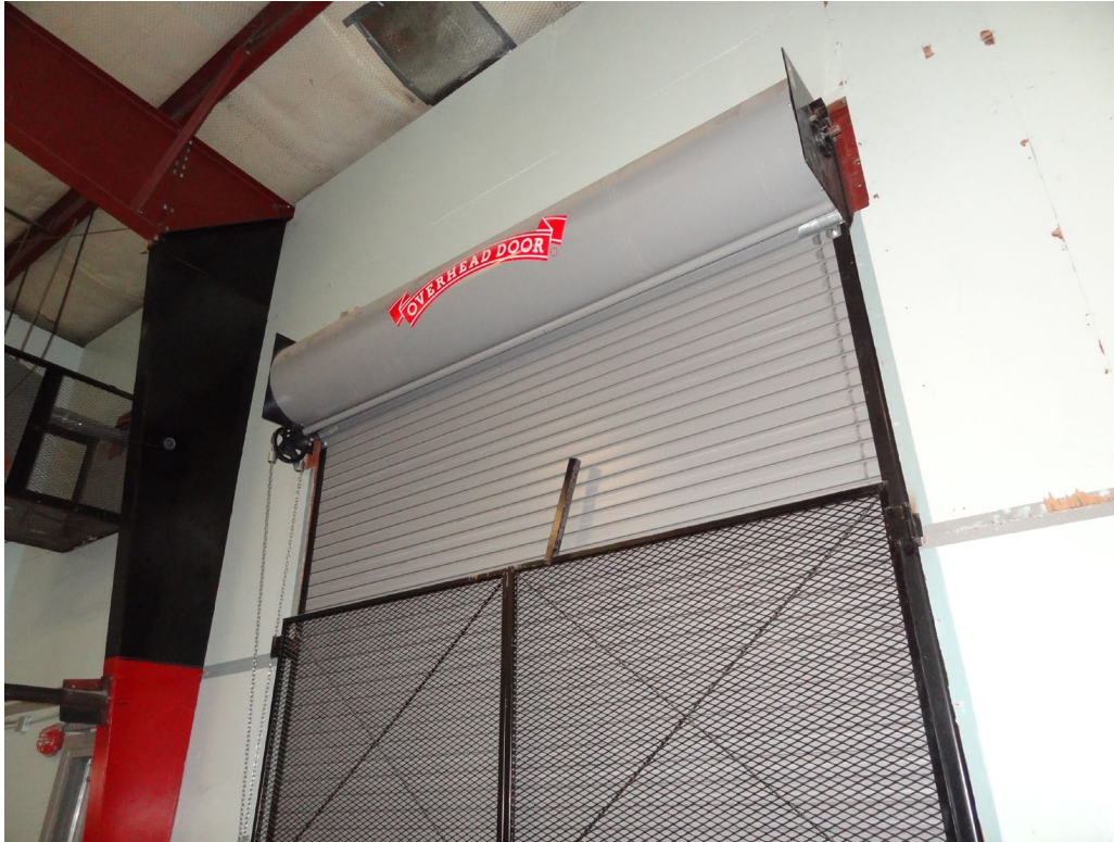
Multi-Purpose / Gymnasium - Building #1389 Description: Replace Overhead Coiling Door.
