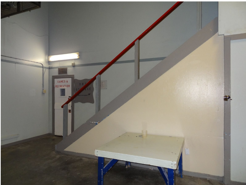
Multi-Purpose / Gymnasium - Building #1389 Description: Rebuild Handrails / Guardrails.
