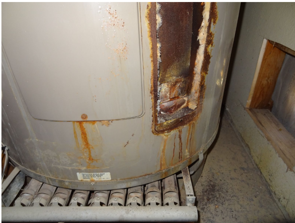
Administration / Housing / Culinary - Building #1388 Description: Replace Water Heaters.
