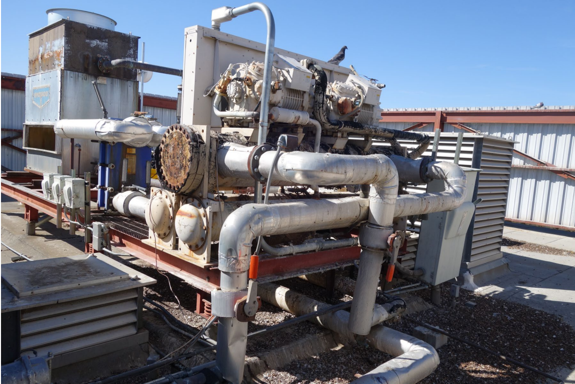
Bradley Building (Vacant) – FCA Building #0266 Description: HVAC System Beyond Useful Life.
