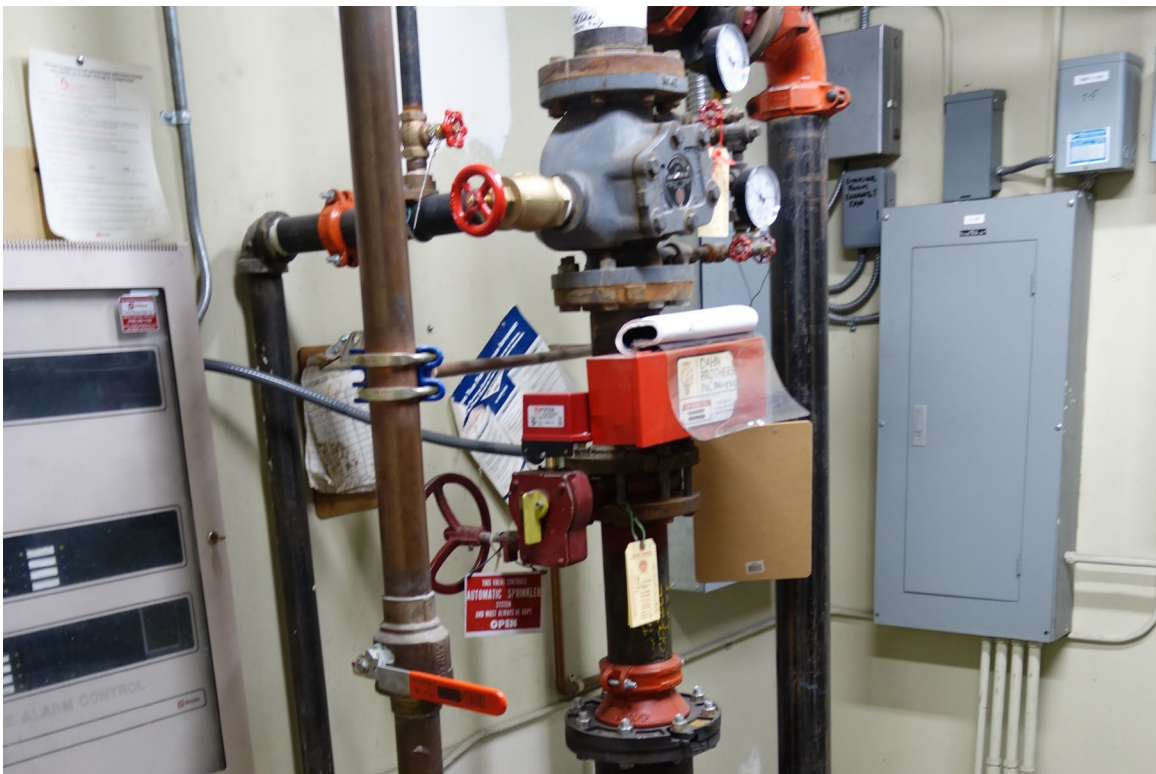
Bradley Building (Vacant) – FCA Building #0266 Description: Fire Riser Reduced Pressure Backflow Needed.
