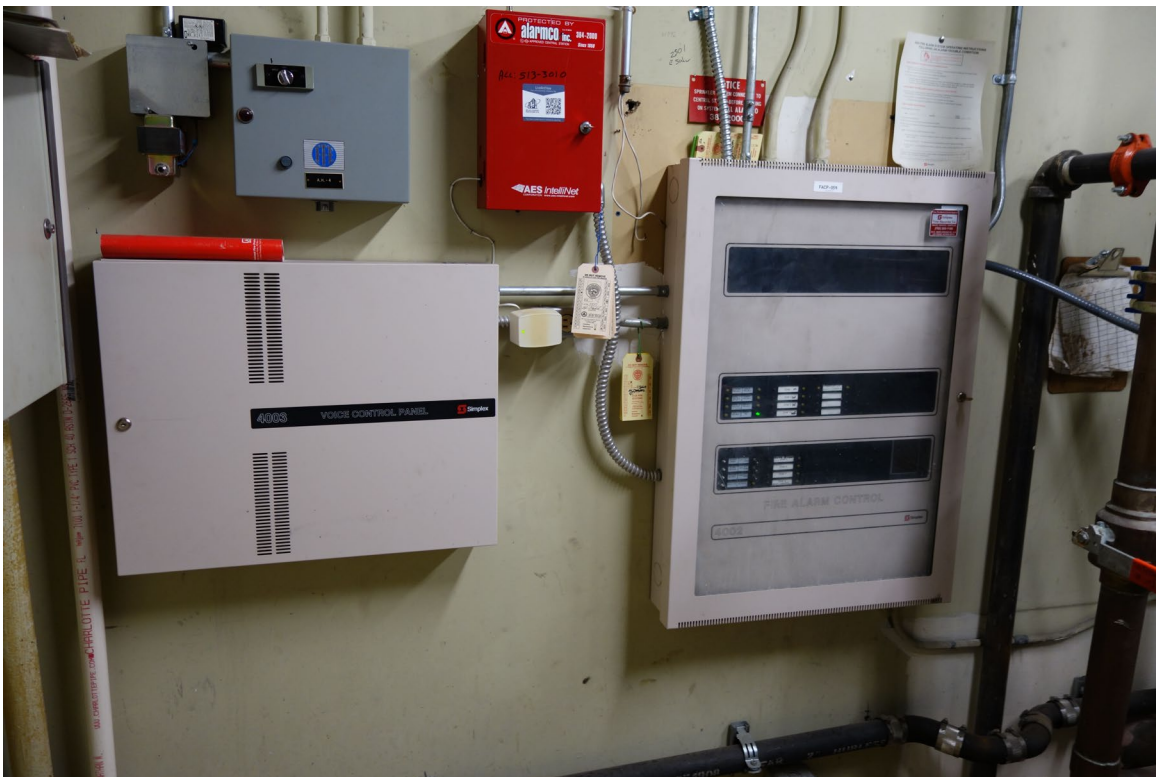
Bradley Building (Vacant) – FCA Building #0266 Description: Fire Alarm System Replacement Needed.
