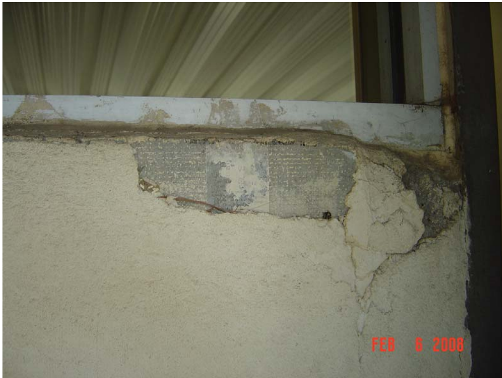
Bradley Building - Building #0266 Description: Damaged stucco at south exit door.
