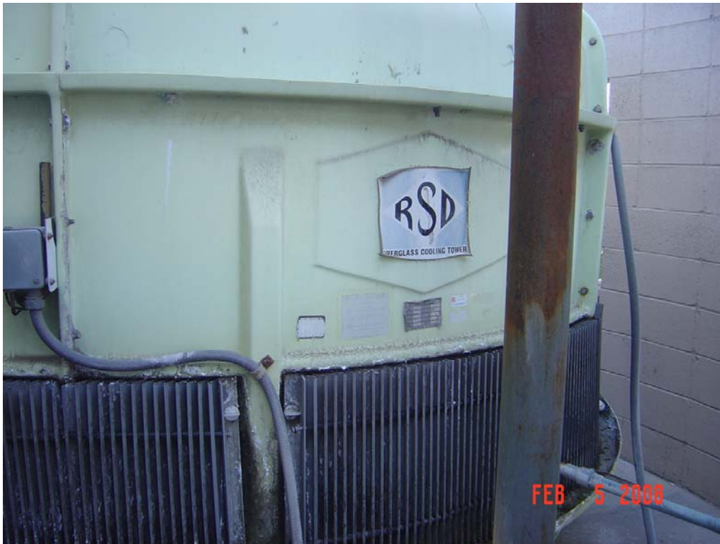
DMV Registration / Inspection Center - Building #0255 Description: Cooling tower.
