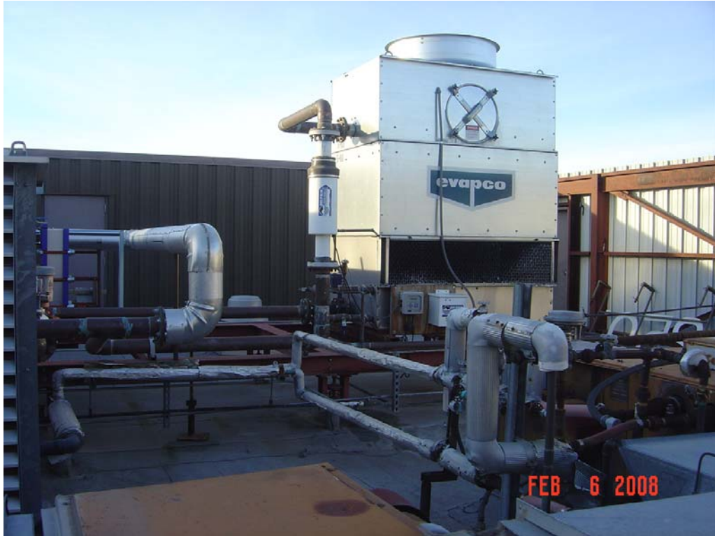
Bradley Building - Building #0266 Description: Cooling tower on the roof.
