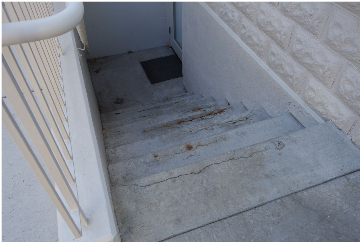
Governor's Mansion - Building #0151 Description: Basement Concrete Stair Replacement Needed.
