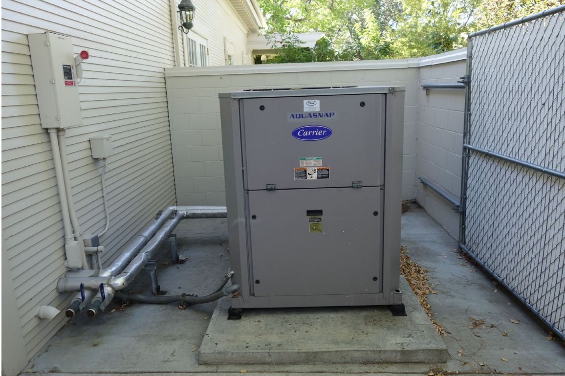
Governor's Mansion Nevada Room - Building #0707 Description: Air Cooled Chiller / HVAC Replacement Plan Recommended.
