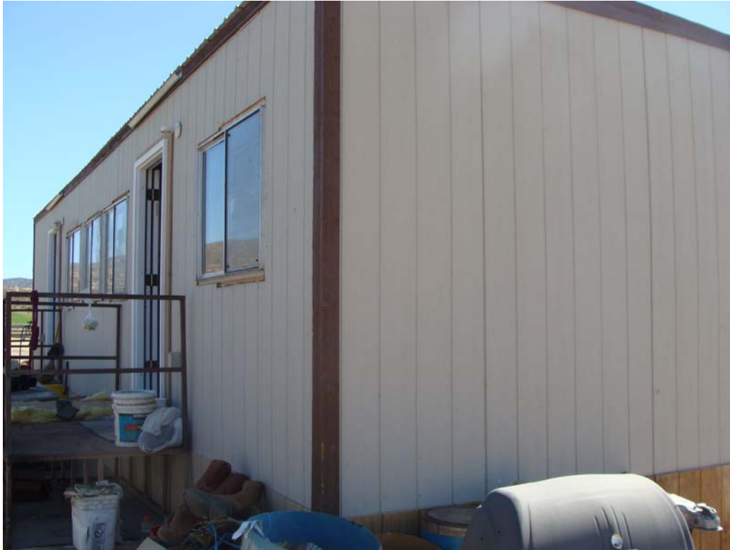
Wild Horse Office - Building #2919 Description: Exterior of the building.
