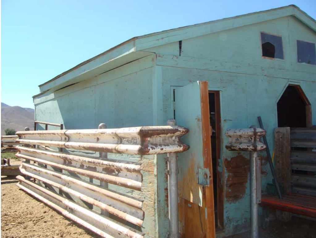
A I Building - Building #2916 Description: Exterior of the building.
