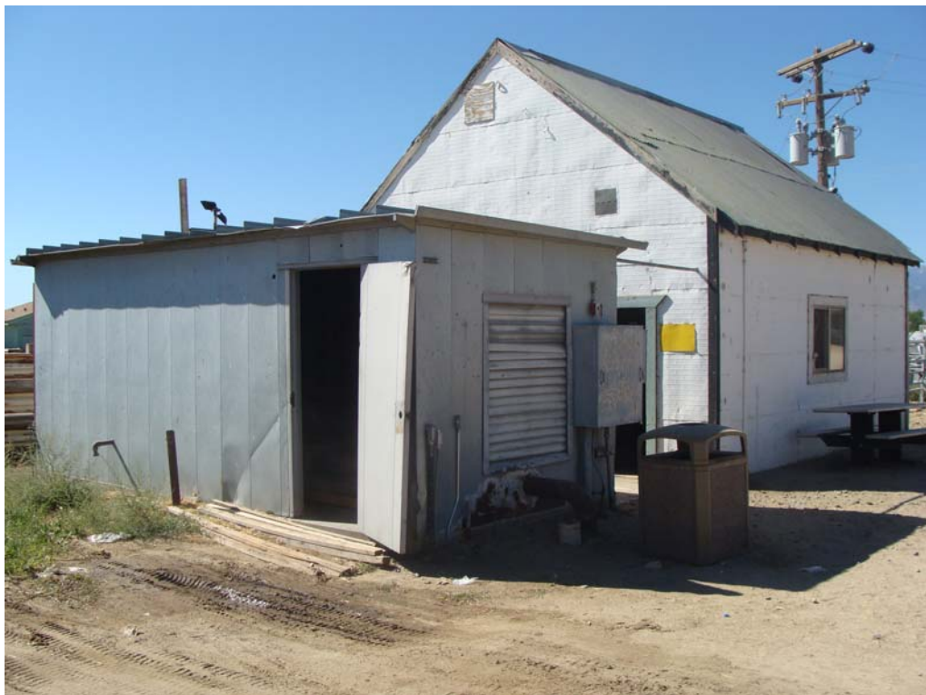
Pump House - Building #0288 Description: Exterior of the building (foreground).
