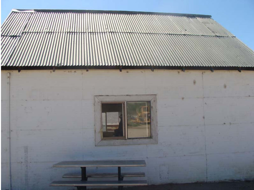
Break Room - Building #0293 Description: Exterior of the building.
