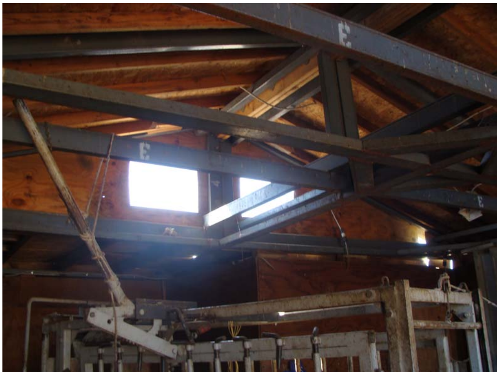
A I Building - Building #2916 Description: Interior of the building.
