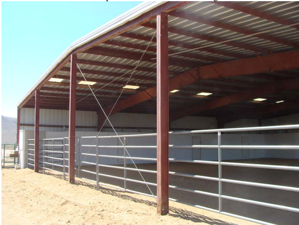
Wild Horse Area - Building #2918 Description: Exterior of the building.
