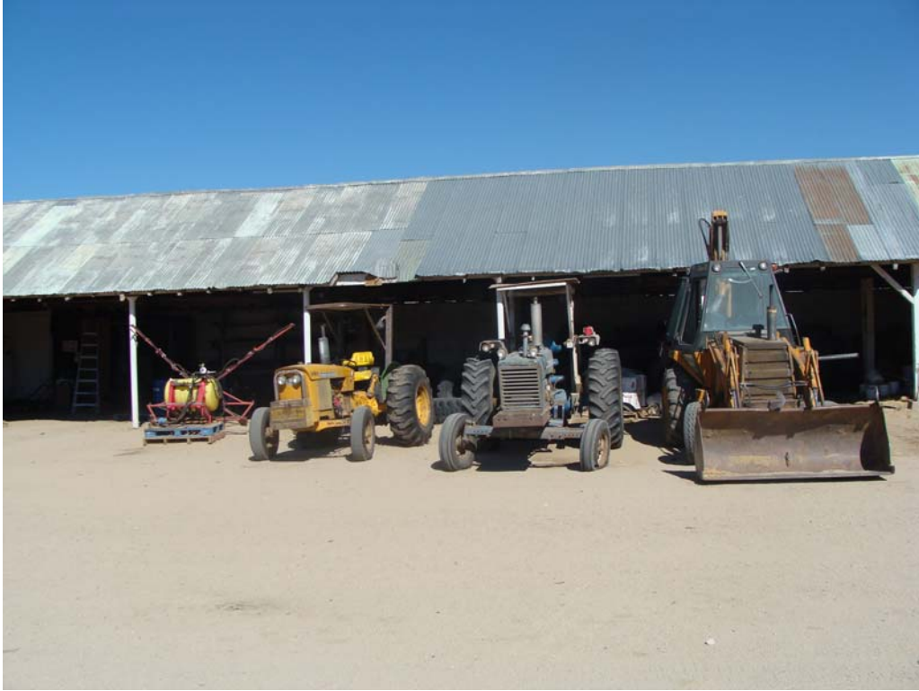
Equipment Shed - Building #1446 Description: East exterior of the building.
