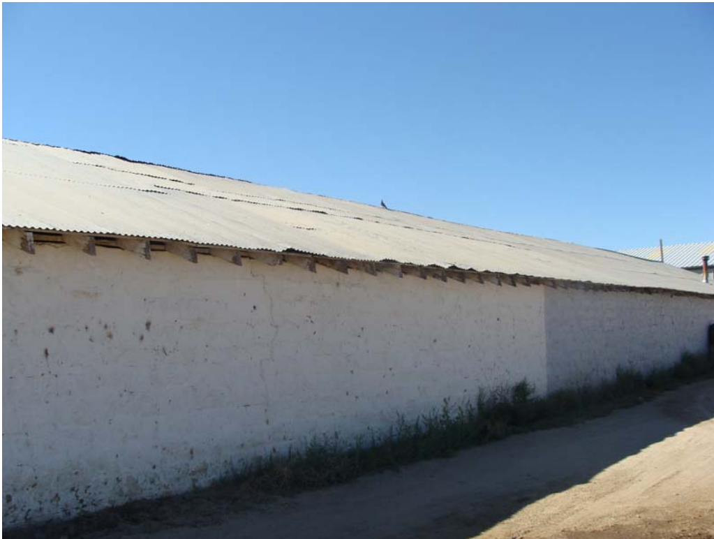
Equipment Shed - Building #1446 Description: West exterior of the building
