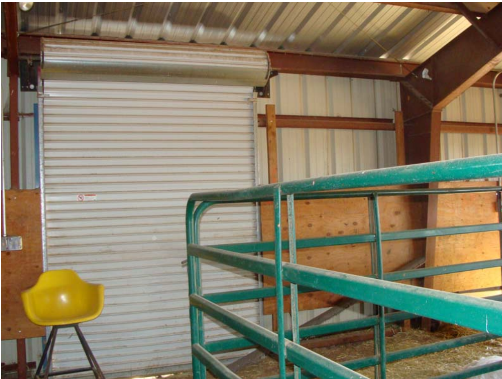
Calving Barn - Building #1447 Description: Interior of the building.
