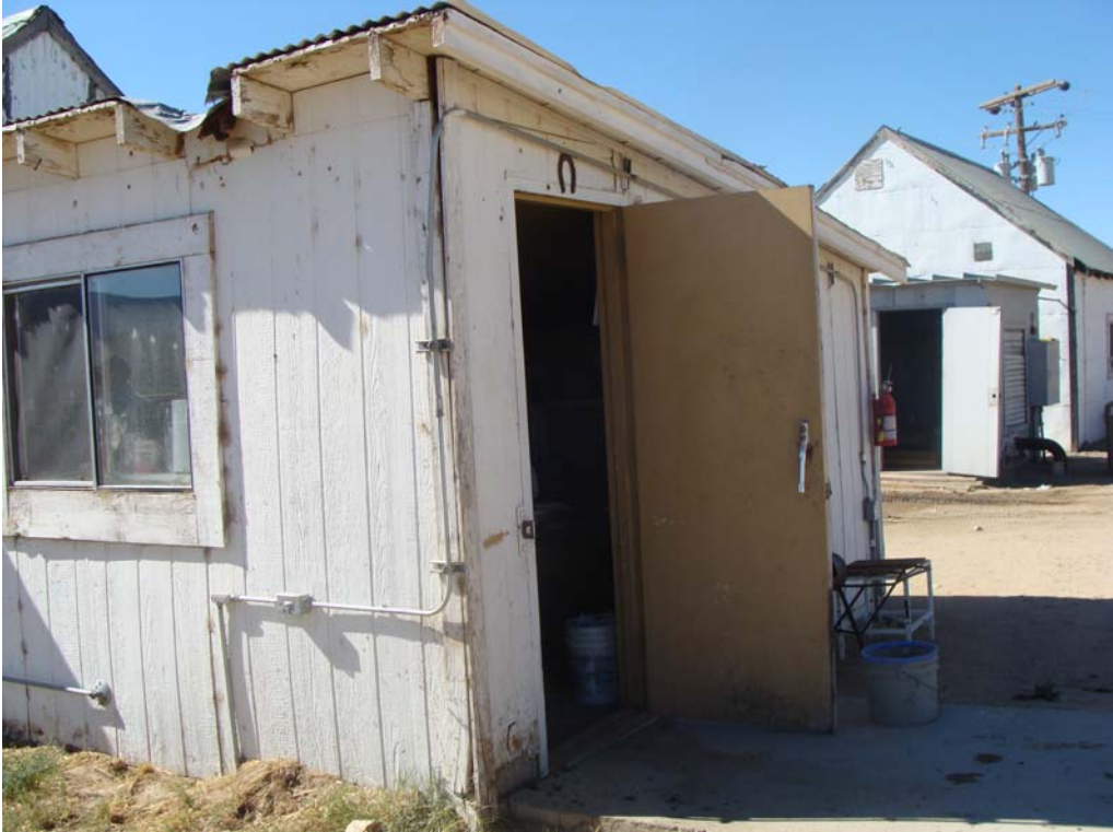
Yard Office - Building #1450 Description: Exterior of the building.
