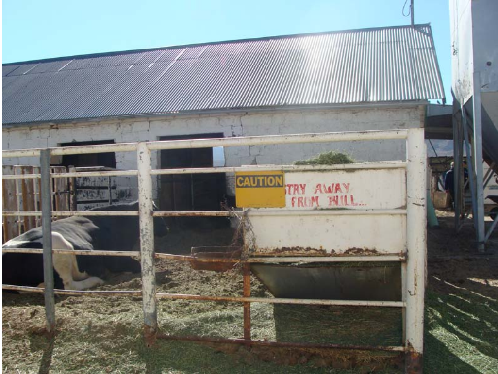
Bull Barn - Building #1440 Description: Exterior of the building.
