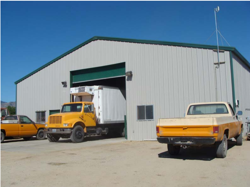
Maintenance Shop - Building #2915 Description: Exterior of the building.
