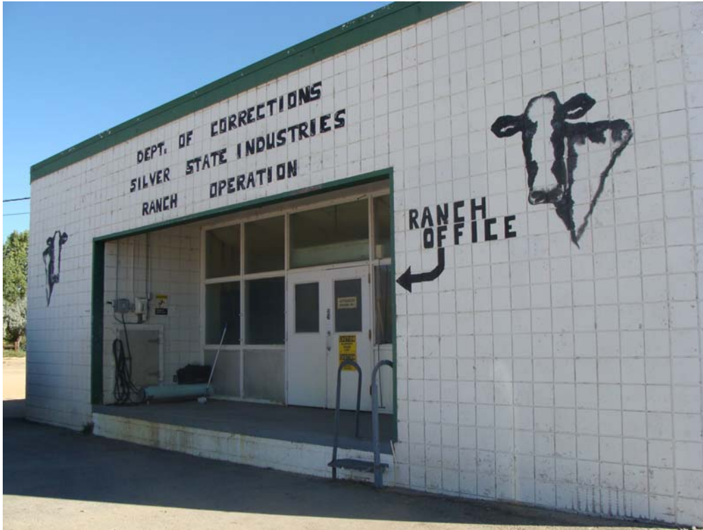
Dairy Barn - Building #1443 Description: Exterior of the building at the loading dock.
