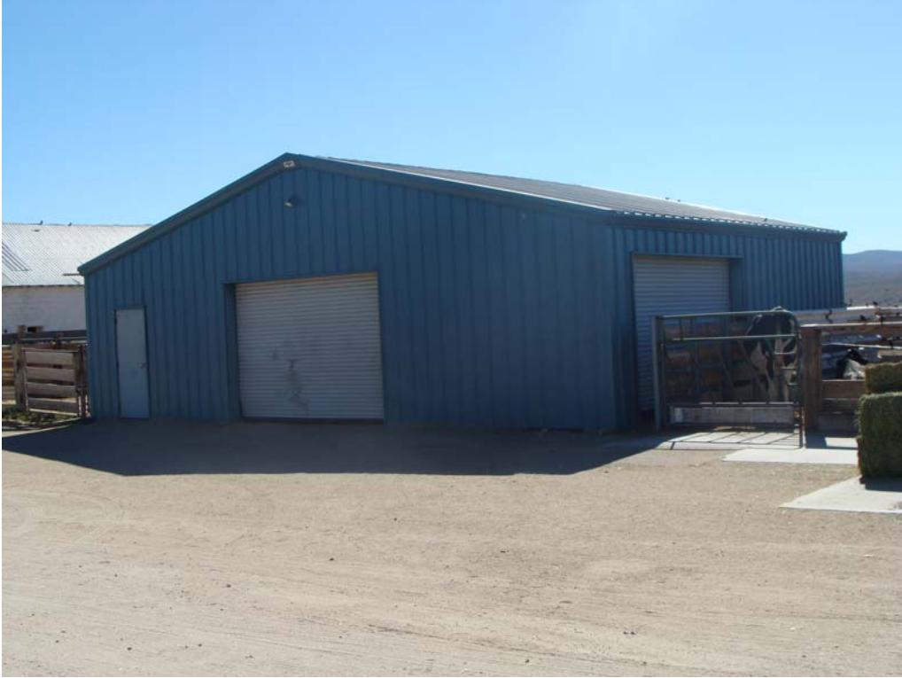
Calving Barn - Building #1447 Description: Exterior of the building.
