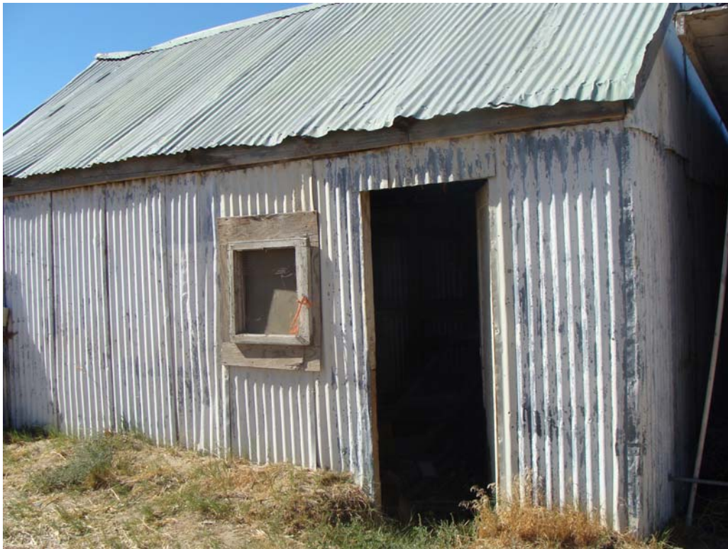
Chicken House - Building #1442 Description: Exterior of the building.
