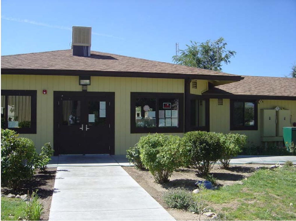
Silver Springs C.C. – Building #0711 Description: The exterior of the Housing Unit
