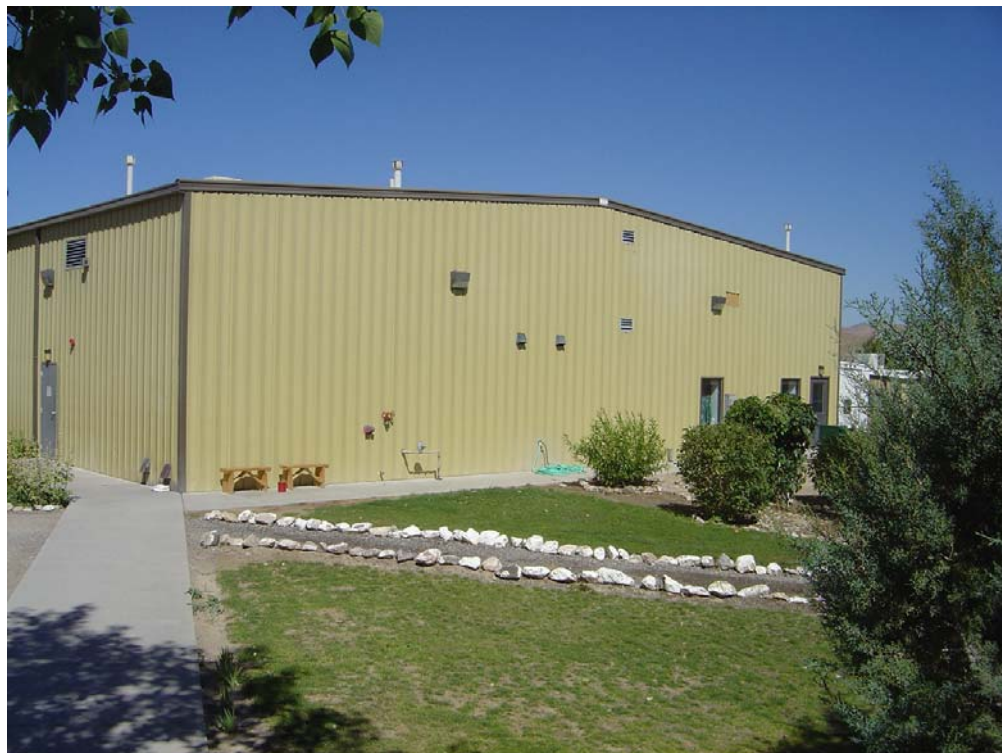
Silver Springs C.C. – Building #1896 Description: The exterior of the Multi-Purpose building
