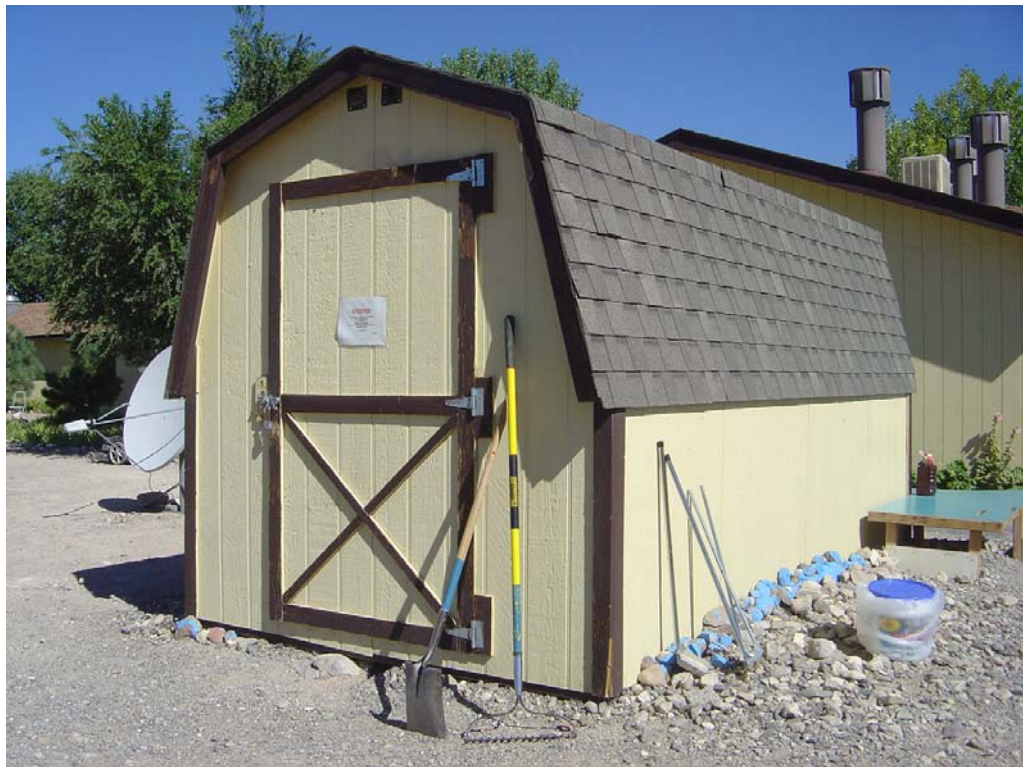
Silver Springs C.C. – Building #2689 Description: Tool Shed
