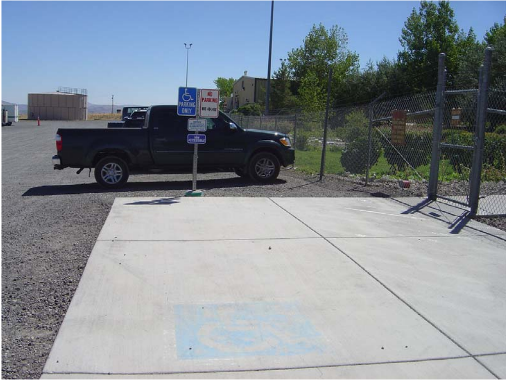
Silver Springs C.C. – Site #9986 Description: ADA accessible parking stall
