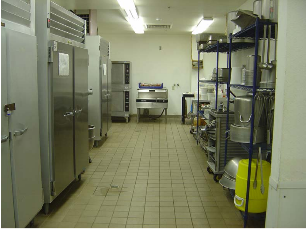
Silver Springs C.C. – Building #1895 Description: The interior of the kitchen
