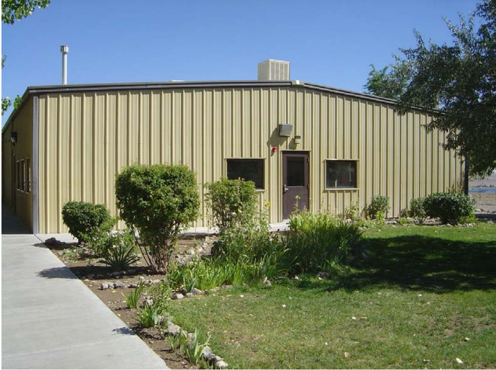
Silver Springs C.C. – Building #1895 Description: The exterior of the Culinary / Dining building
