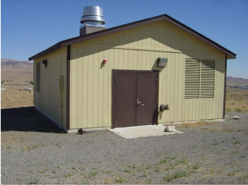
Silver Springs C.C. – Building #2029 Description: Generator Building
