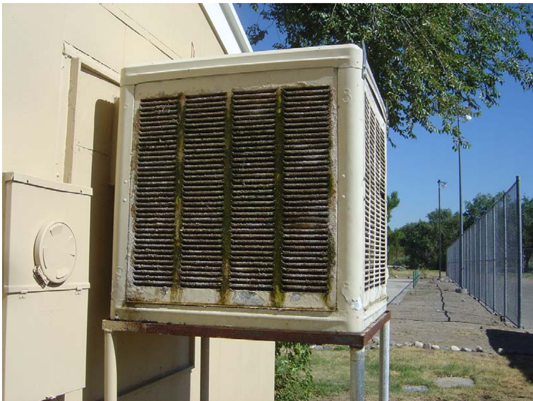
Northern Nevada Restitution Center – Building #1895 Description: Evaporative cooler is extremely scaled
