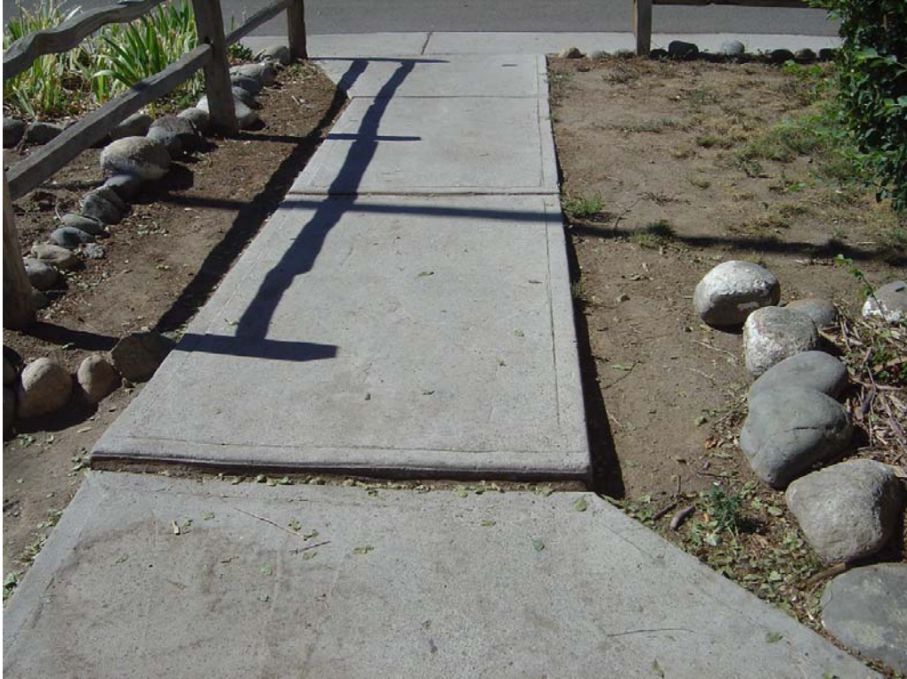
Northern Nevada Restitution Center – Building #1487 Description: Sidewalk heaving at entrance to Culinary building
