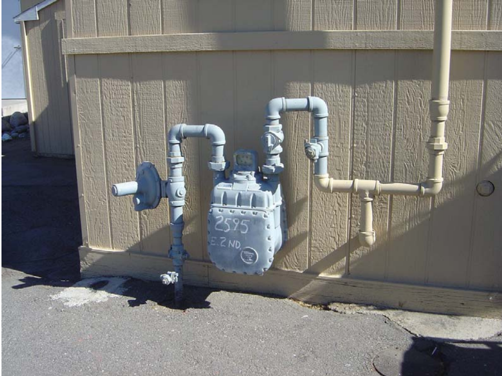
Northern Nevada Restitution Center – Building #1484 Description: Need to install a Seismic Gas Shut Off
