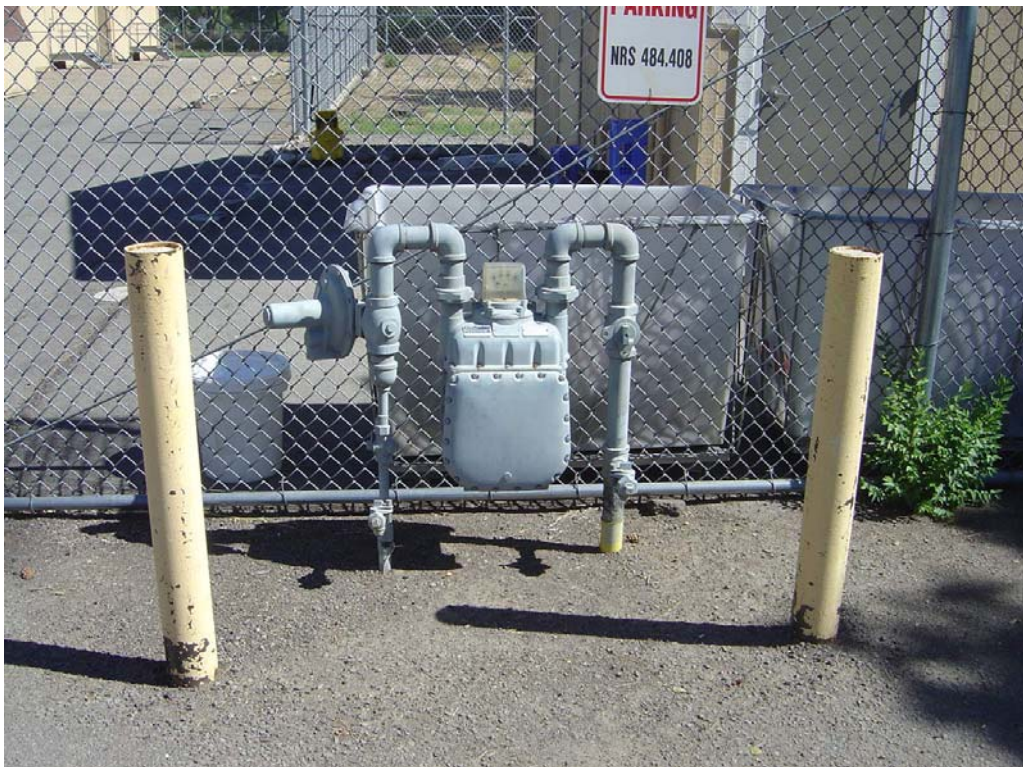
Northern Nevada Restitution Center – Site #9987 Description: Need to install a Seismic Gas Shut Off Valve
