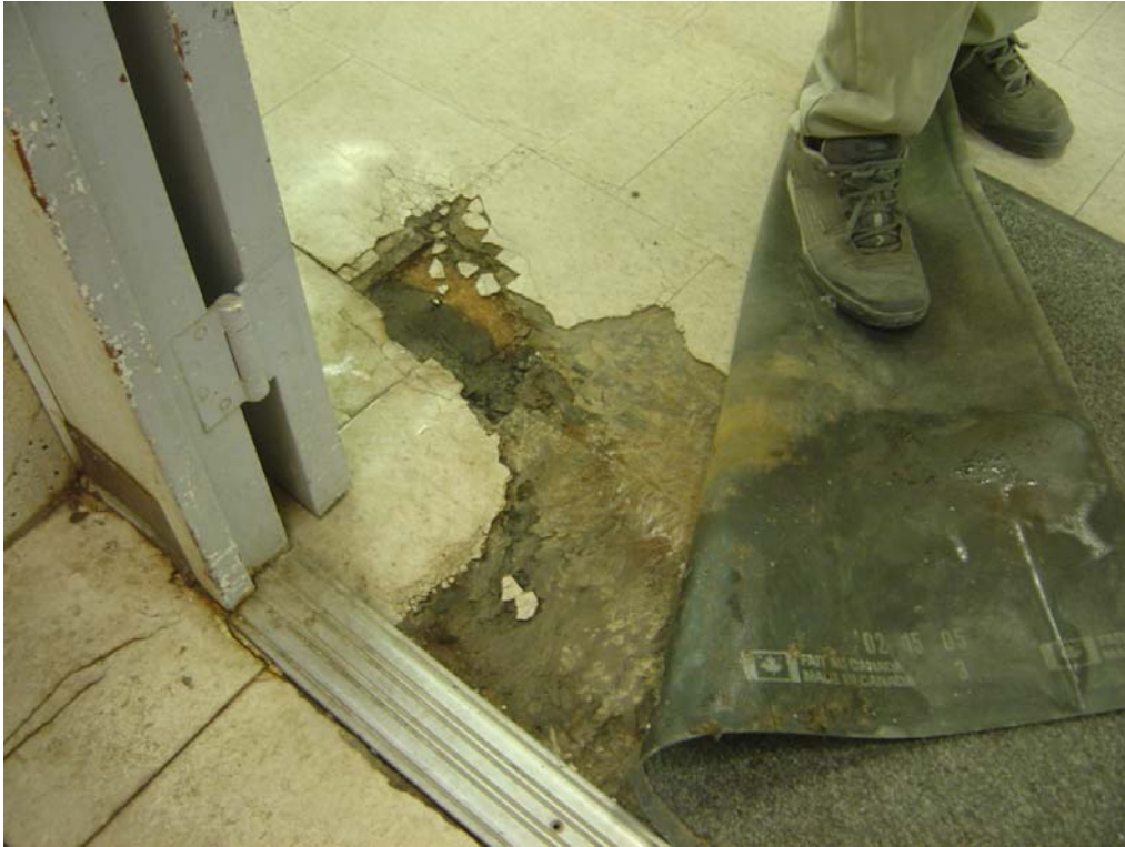
Northern Nevada Restitution Center – Building #1484 Description: Damaged sub flooring
