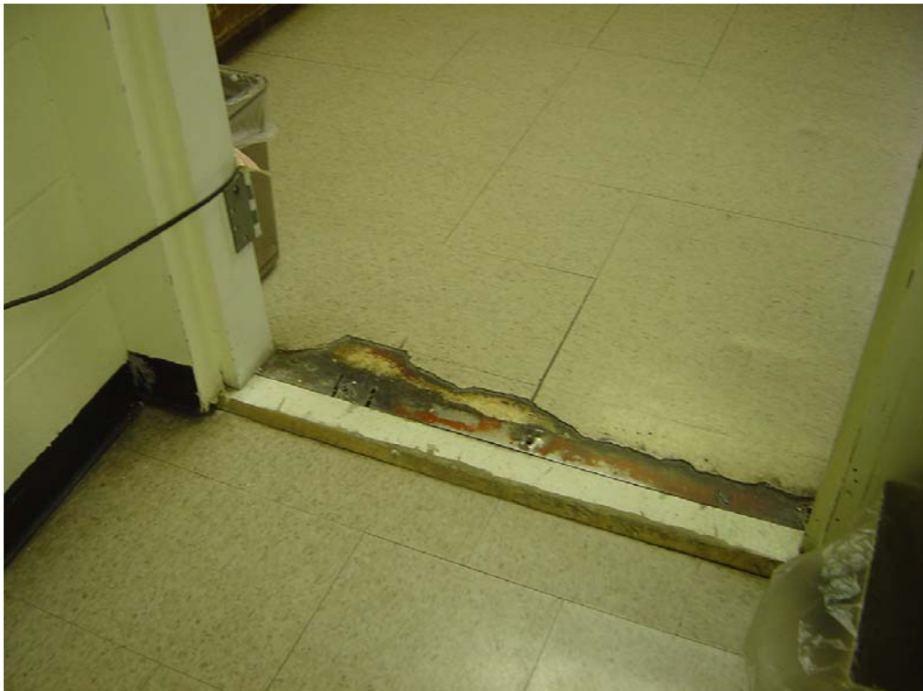
Northern Nevada Restitution Center – Building #1484 Description: Interior view of damaged VCT
