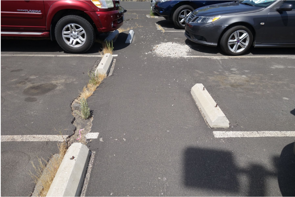
Warm Springs Correctional Center Site – FCA Site #9988 Description: Patch, Crack & Slurry Seal Asphalt Paving.
