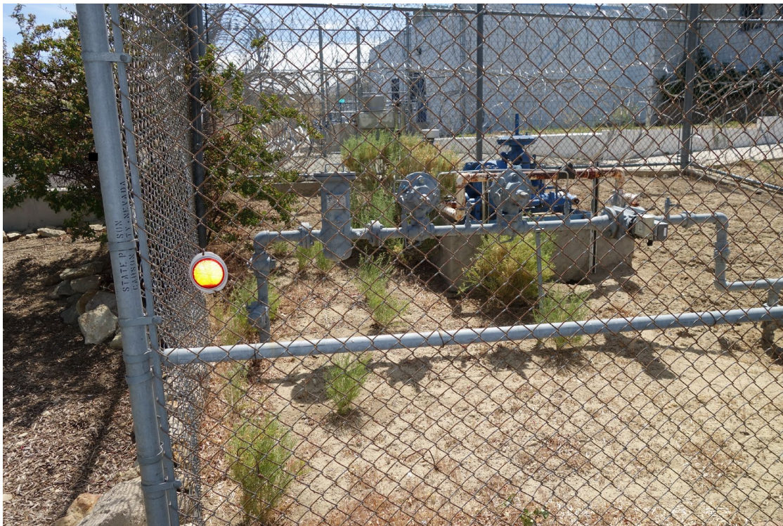
Warm Springs Correctional Center Site – FCA Site #9988 Description: Seismic Gas Shut-Off Valve Needed.
