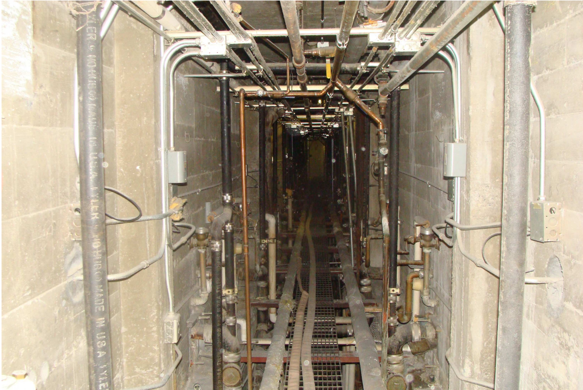
Administration/ Cell Blocks - Building #0094 Description: Typical pipe chase in Cell Blocks.
