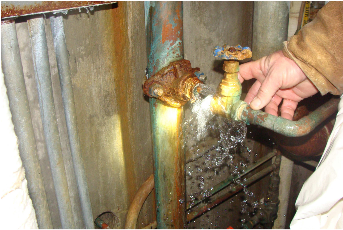
Administration/ Cell Blocks - Building #0094 Description: Example of broken domestic water line in Cell Block Unit 5.
