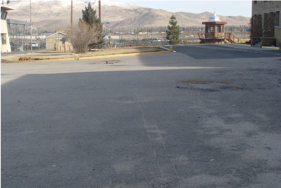
Nevada State Prison - Site #9989 Description: Asphalt in need of repair and sealing.
