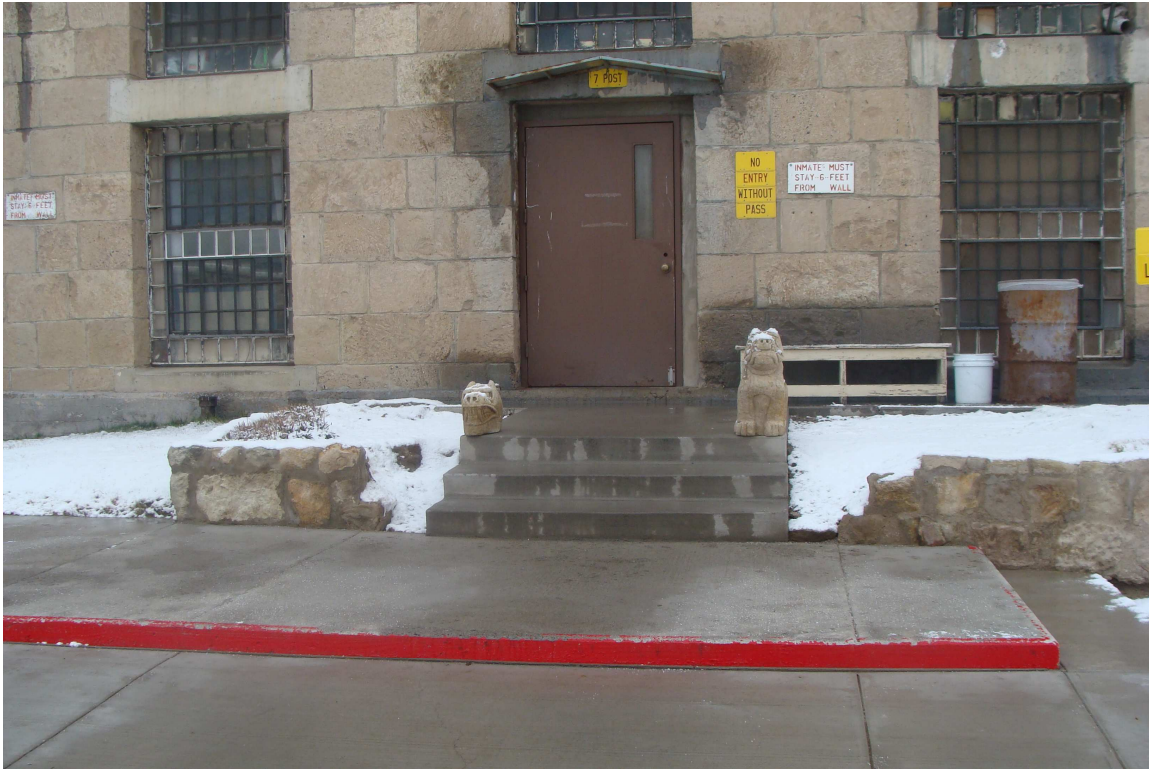
Nevada State Prison - Site #9989 Description: Existing stairs in need of handrails.
