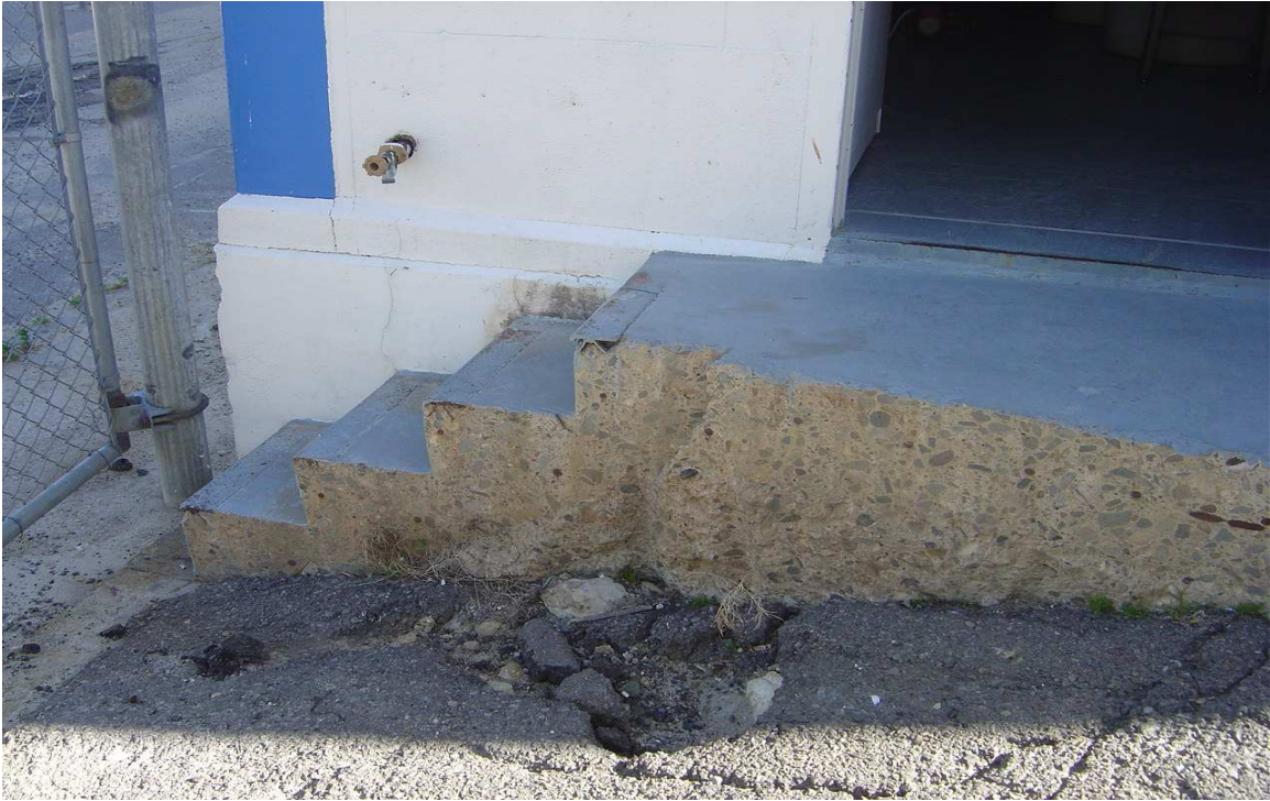
Boiler Plant - Building #0099 Description: Exterior stairs in need of replacement.
