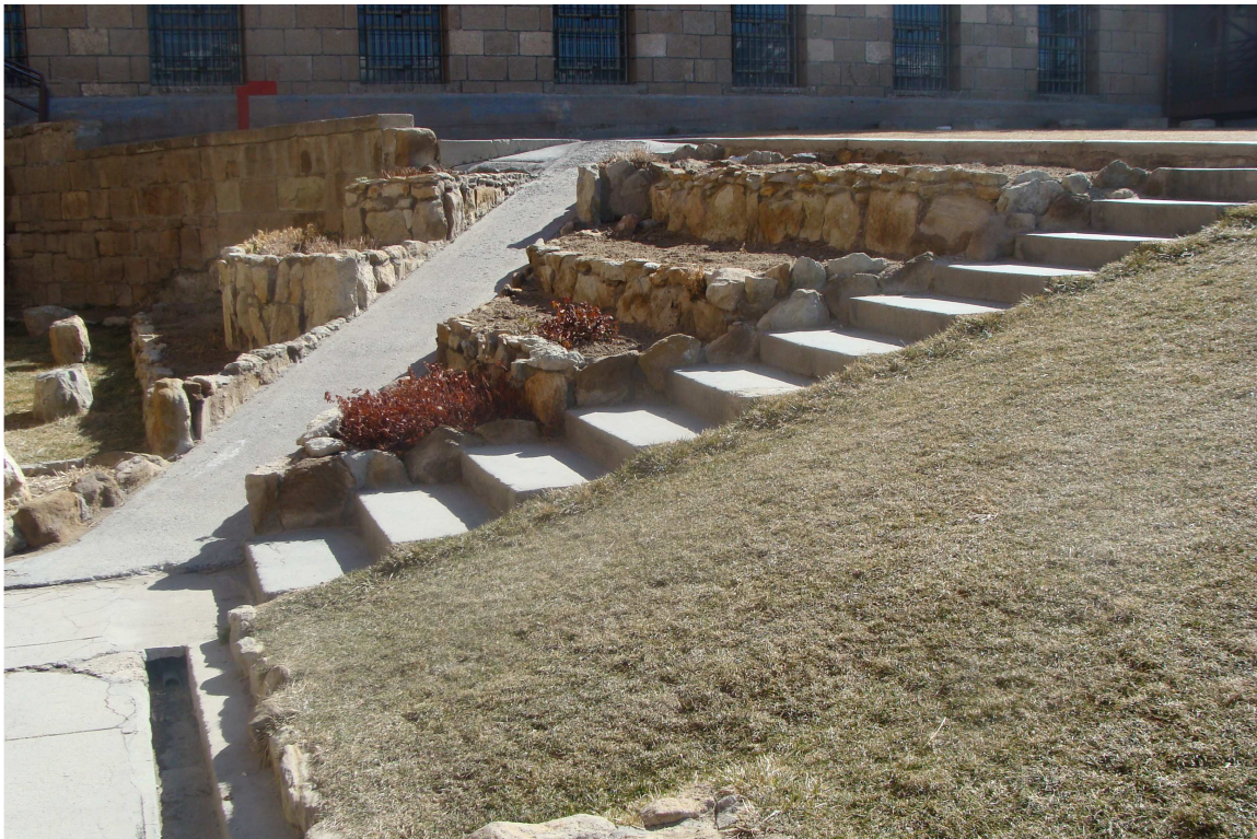
Nevada State Prison - Site #9989 Description: Lower yard stairs in need of handrails.
