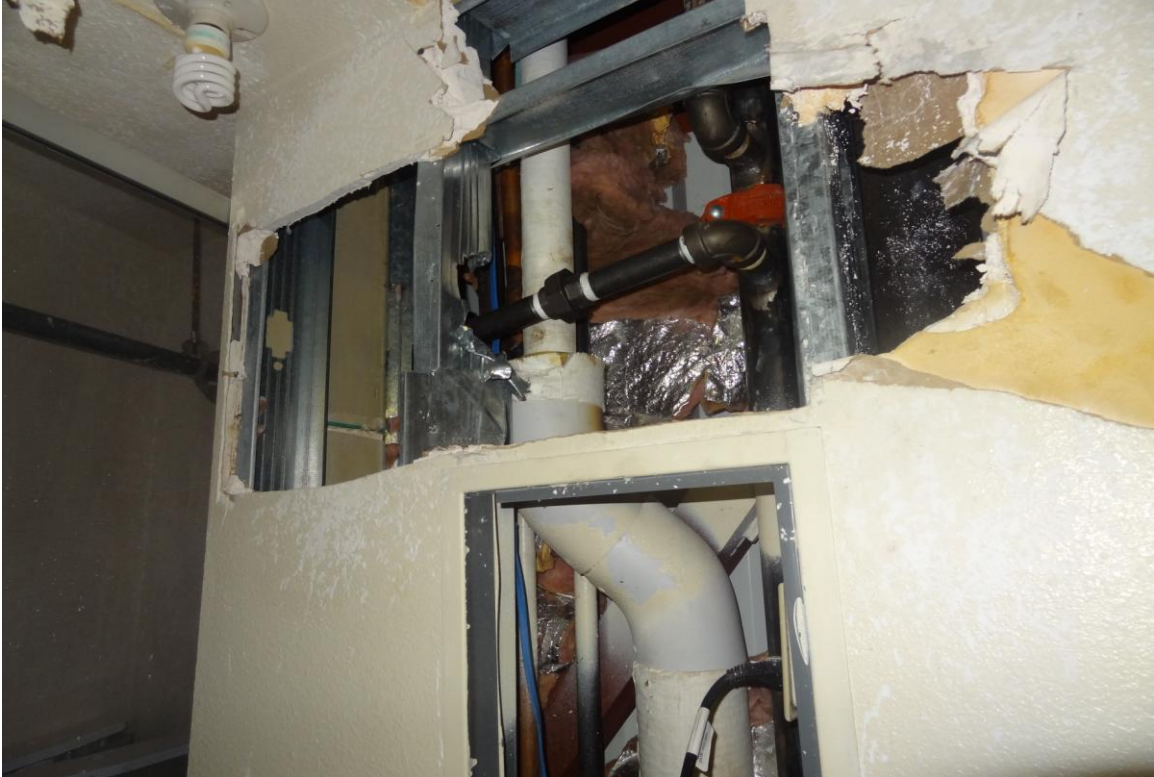
Guard Tower 3 – FCA Building #0146 Description: Water damage to the interior.
