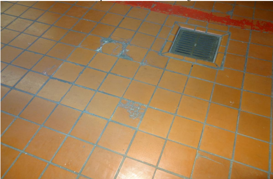
Culinary / Dining – FCA Building #0129 Description: Culinary floor in need of replacement.
