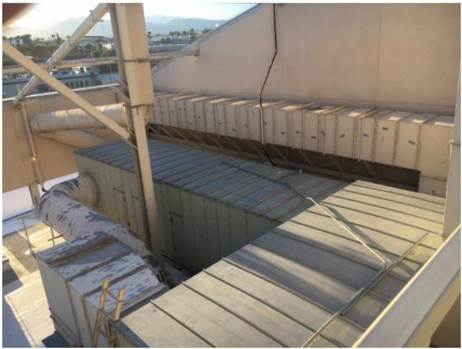
5 - HVAC Ductwork on Roof
