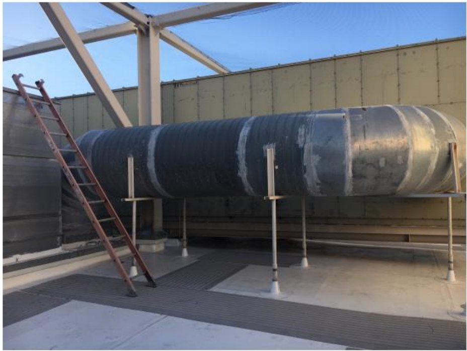
1 - HVAC Ductwork on Roof
