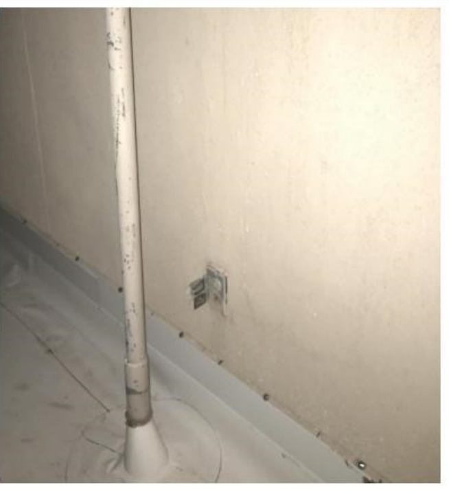
5 - Receptacles in wet locations exposed to sky are left open. Suggest replacing with "while-in-use" covers.
