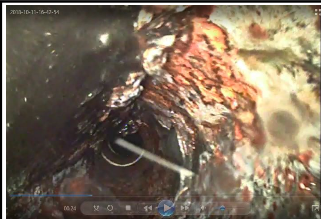
1 - Plumbing Systems - Underground - Collapsed Cast Iron
