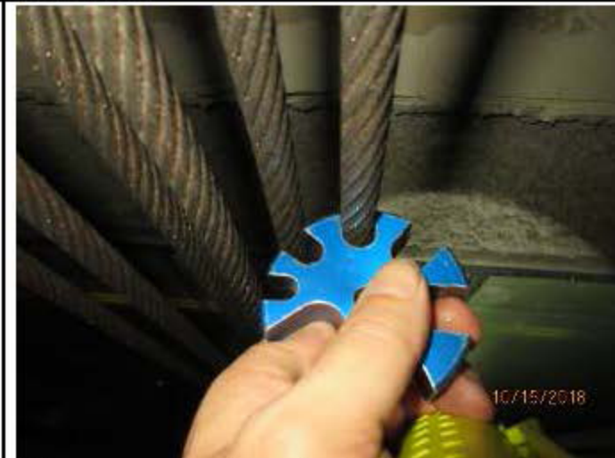
Hoist ropes are rouging and undersized, require replacement.
