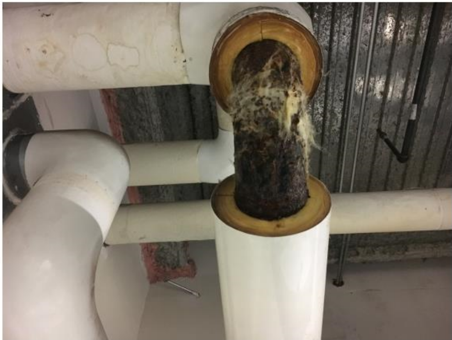
4 - Hydronic Piping - Exterior Corrosion & Insulation
