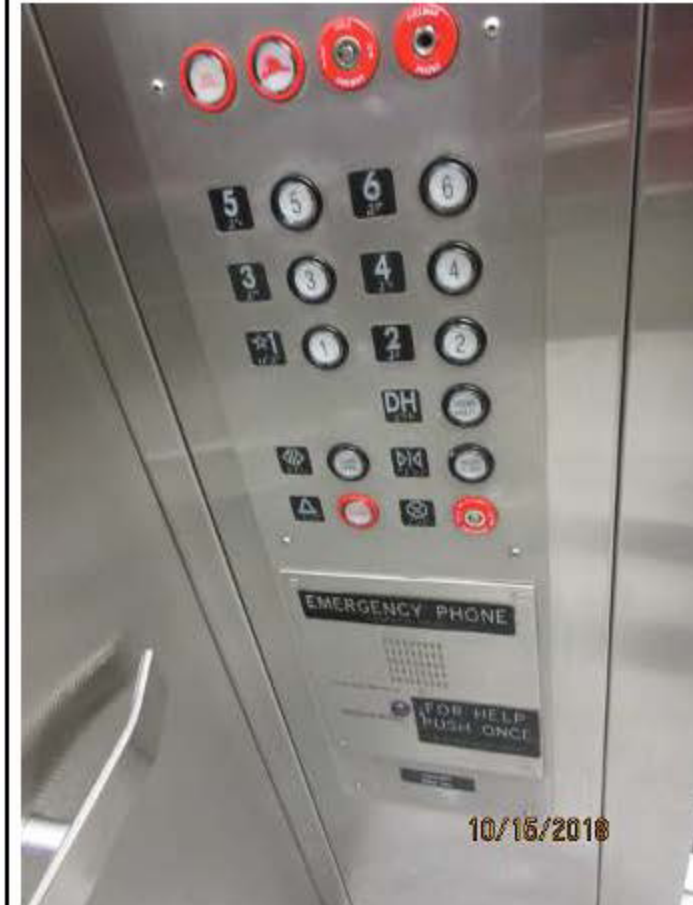
Car panel is ADA compliant and in good condition.
