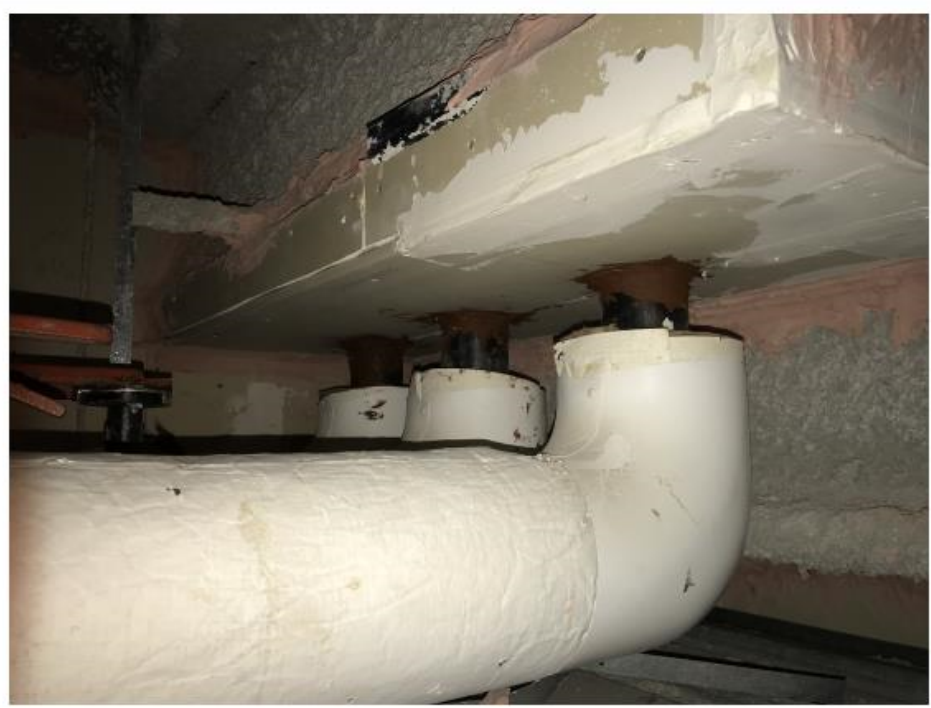
5 - Hydronic Piping - Exterior Condition & Insulation
