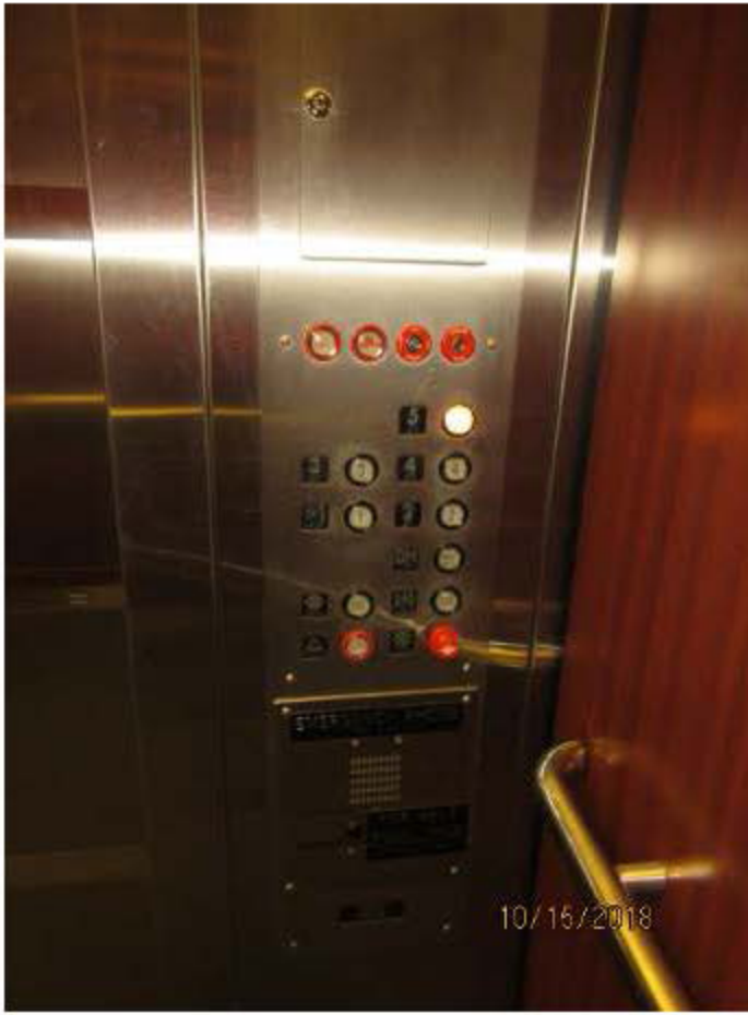
Typical car operating panel
