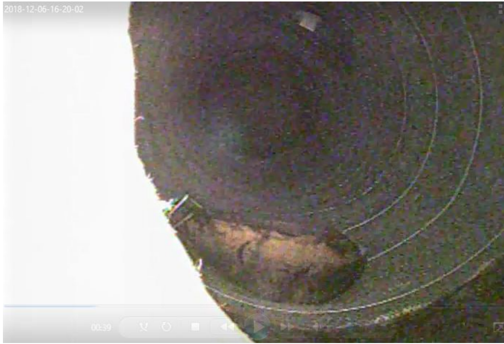
3 - Duct Section - Fitting Penetration - Exposed Fiberglass
