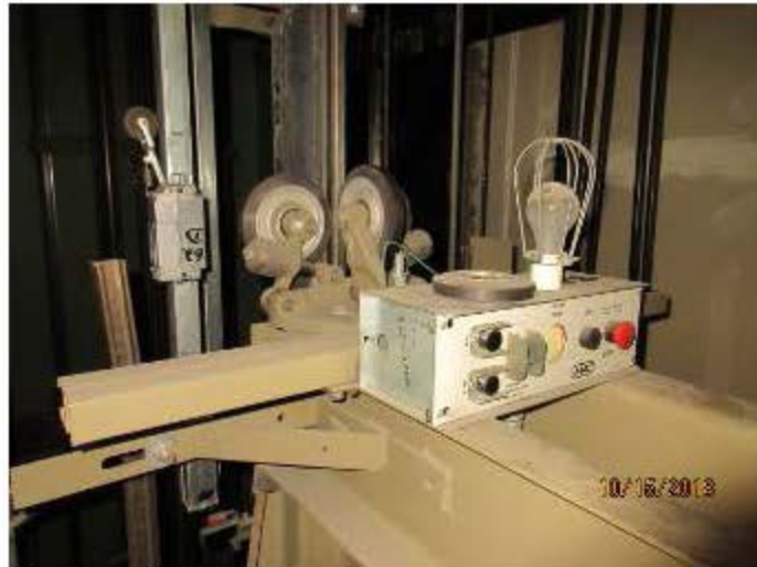
Top of car inspection station.
