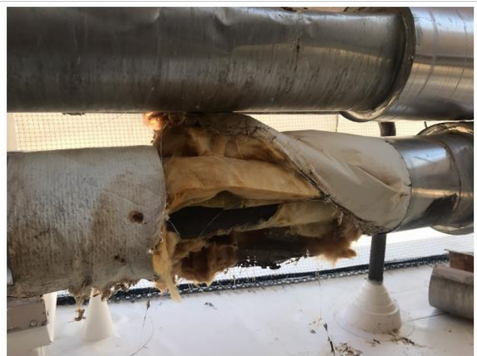
6 - Hydronic Piping - Exterior Corrosion & Insulation
