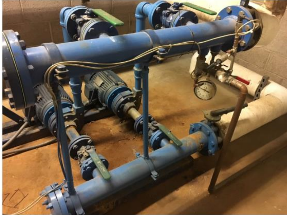
2 - Plumbing Systems - Domestic Booster Pump
