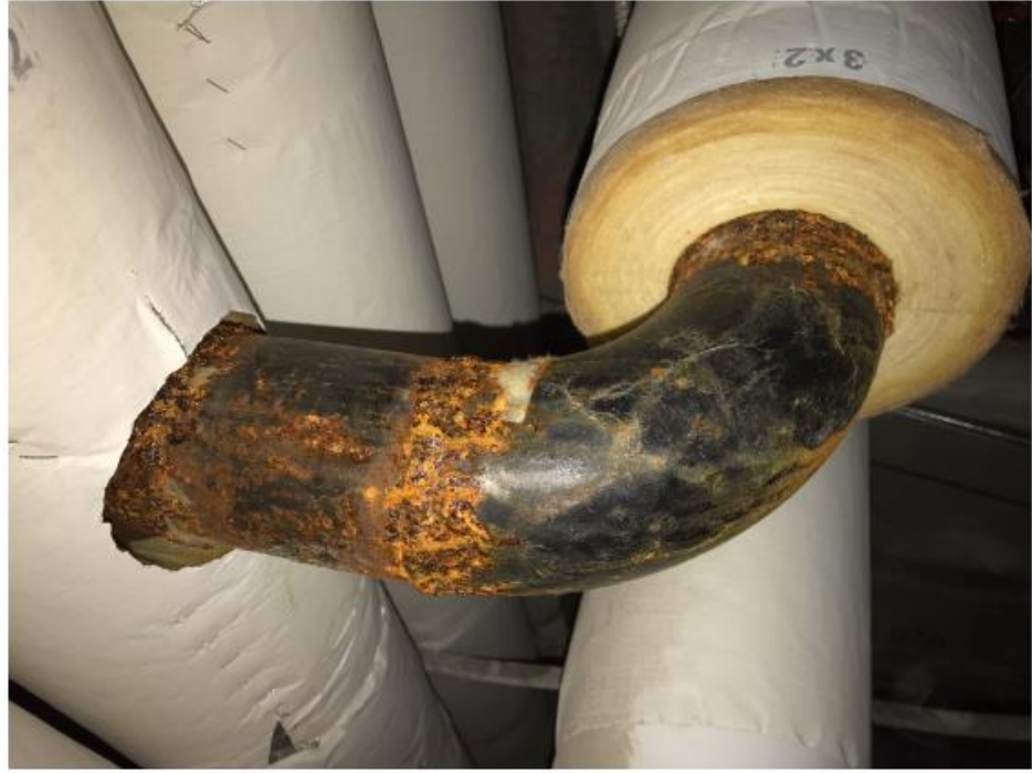
2 - Hydronic Piping - Exterior Condition & Insulation
