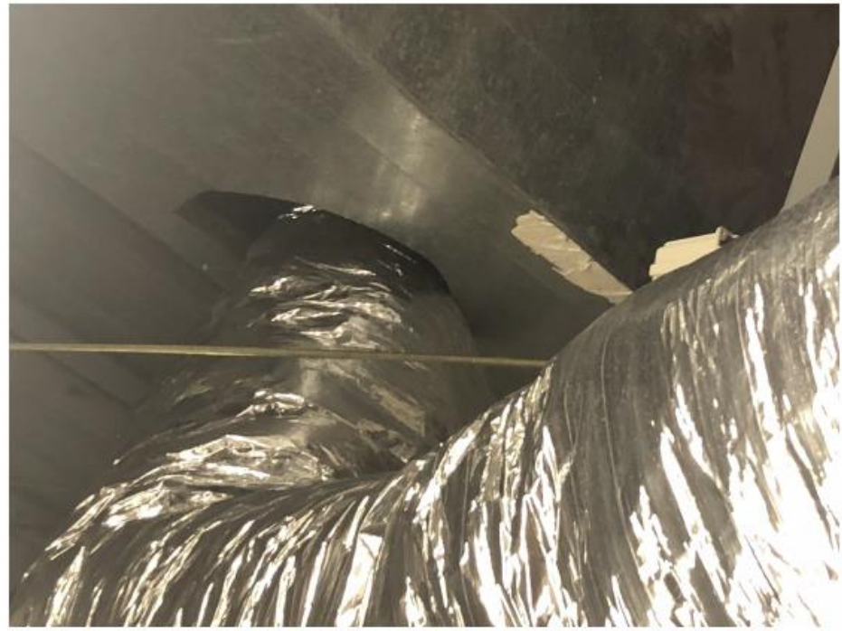
4 - HVAC Flexible Ductwork
