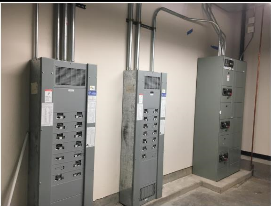
2 - Emergency dist. boards 'EDP2' (left) and 'EDP3' (center) are installed with incorrect rating. 250A equipment connected to 600A feeders.
