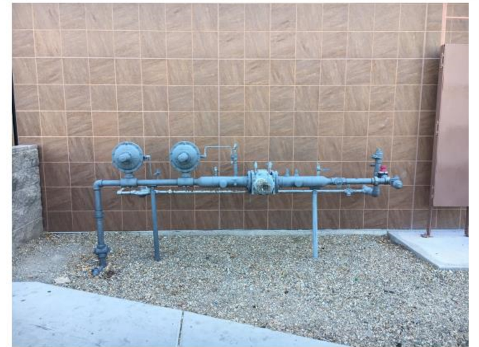
6 - Plumbing Systems - Gas Meter
