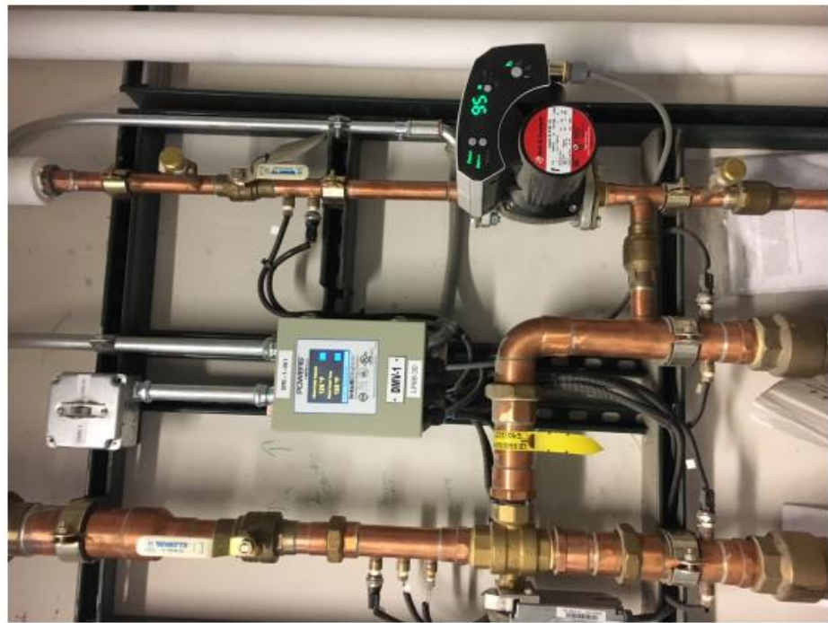
4 - Plumbing Systems - Tempering Station
