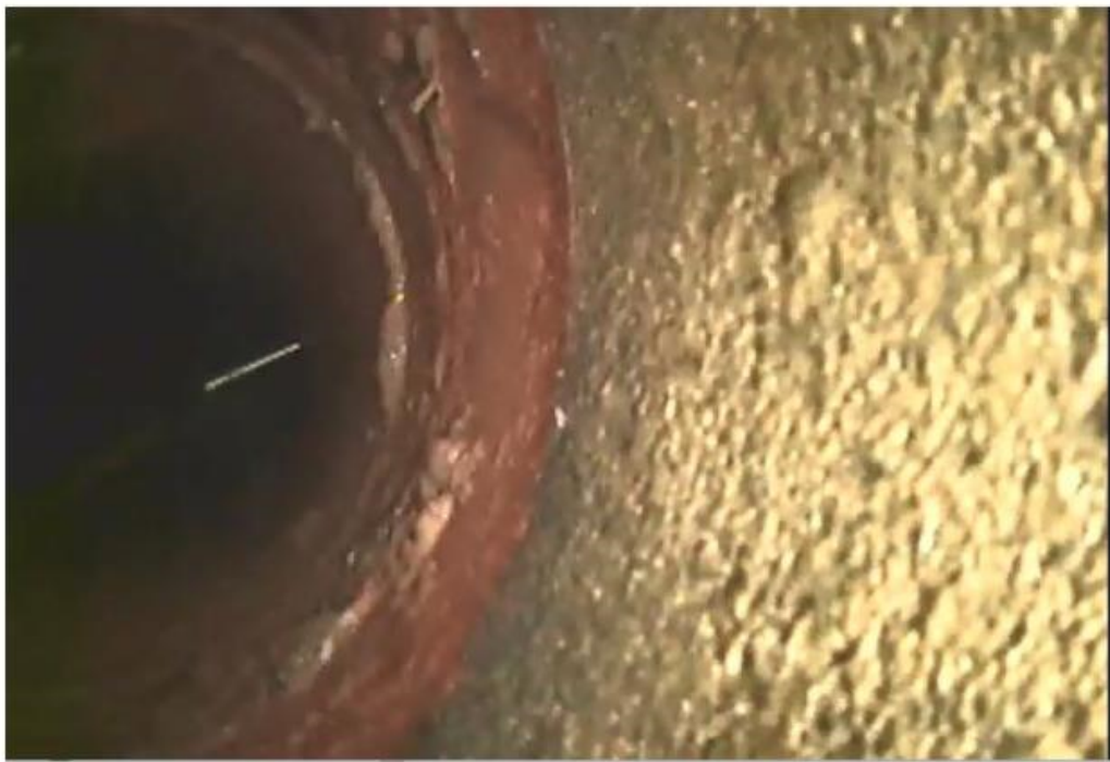
4 - Hydronic Piping - Interior Condition
