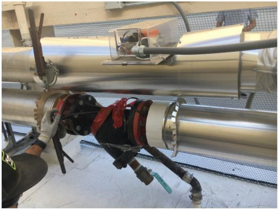
6 - Hydronic Piping - Camera Insertion Point
