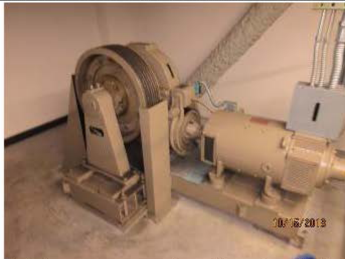
Typical passenger worm and gear DC machine with DC motor.
