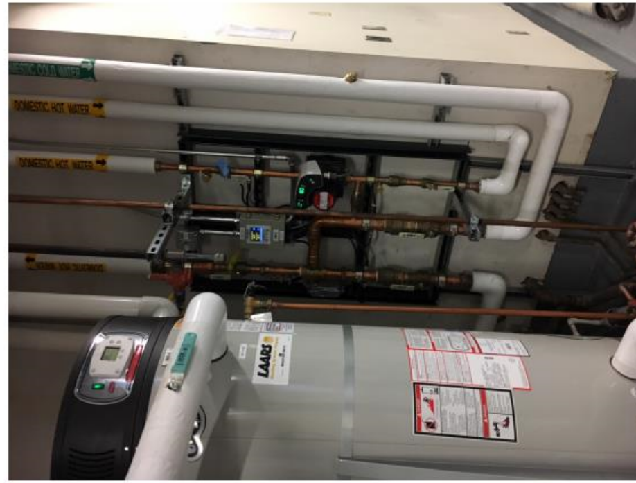
2 - Plumbing Systems - Tempering Station
