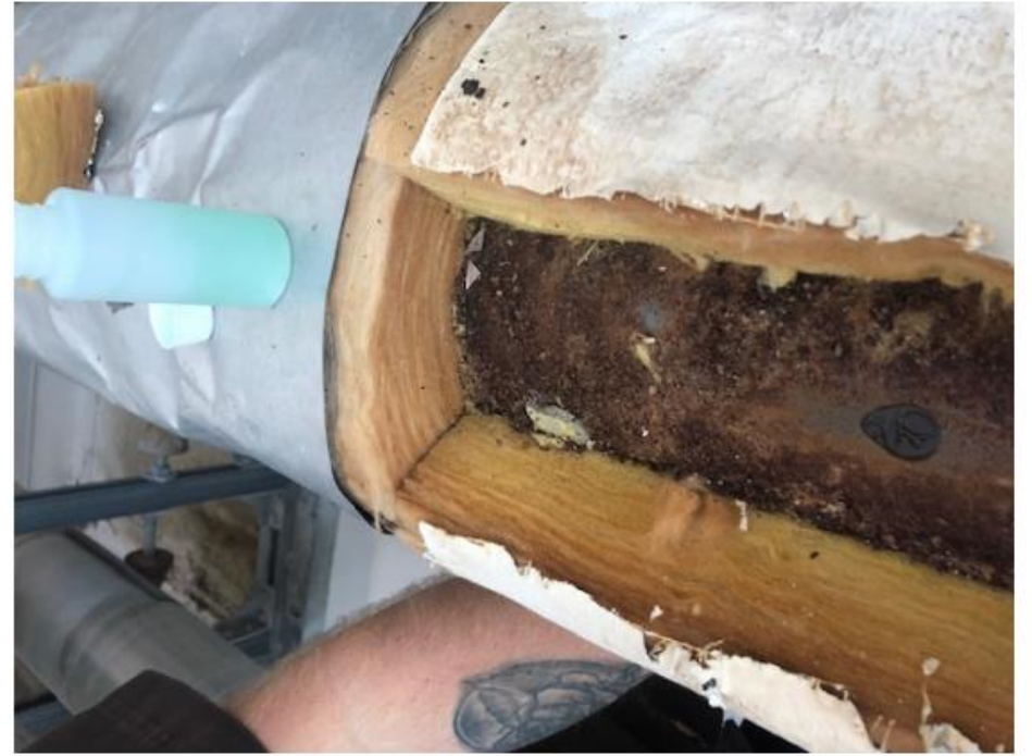
3 - Hydronic Piping - Exterior Corrosion & Insulation
