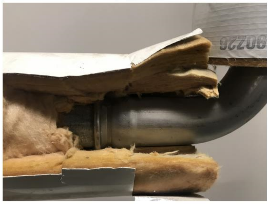
2 - Hydronic Piping - Heating Hot Water
