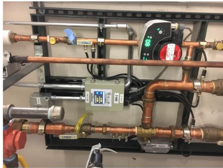
5 - Plumbing Systems - Tempering Station
