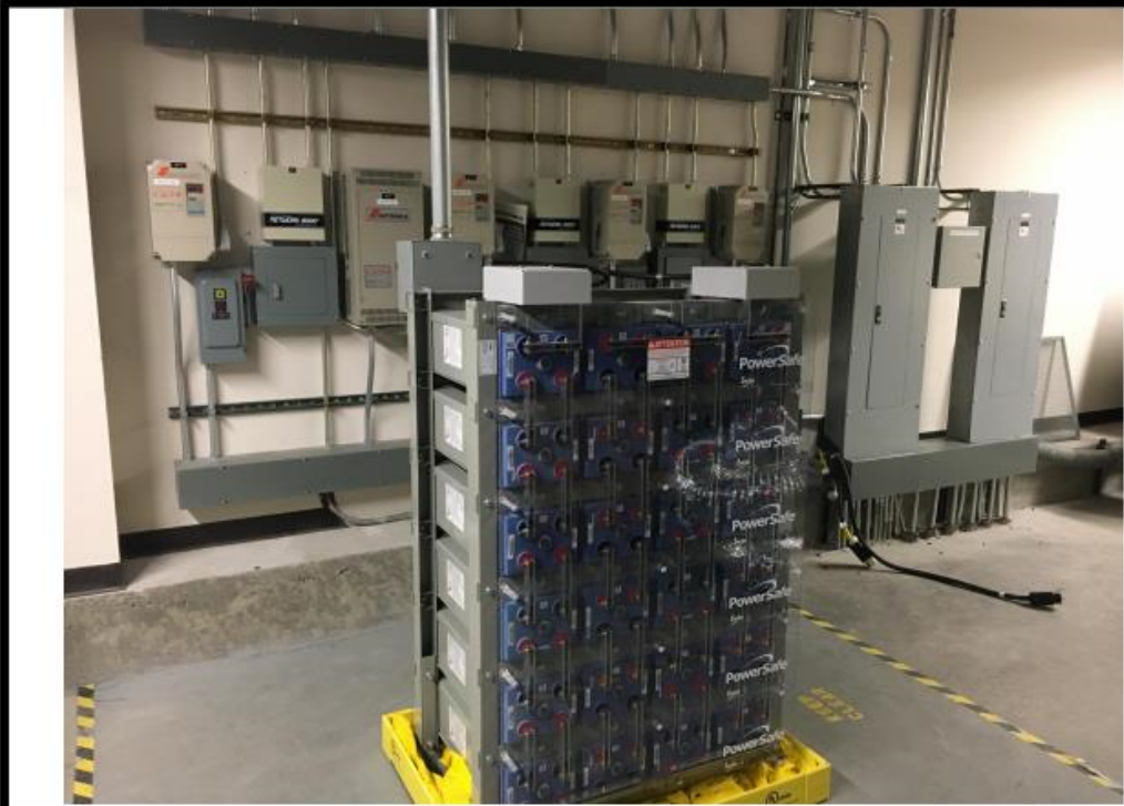
1 - String of VRLA batteries located in the Level 6 electrical room.
