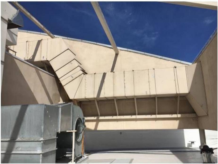
6 - HVAC Ductwork on Roof
