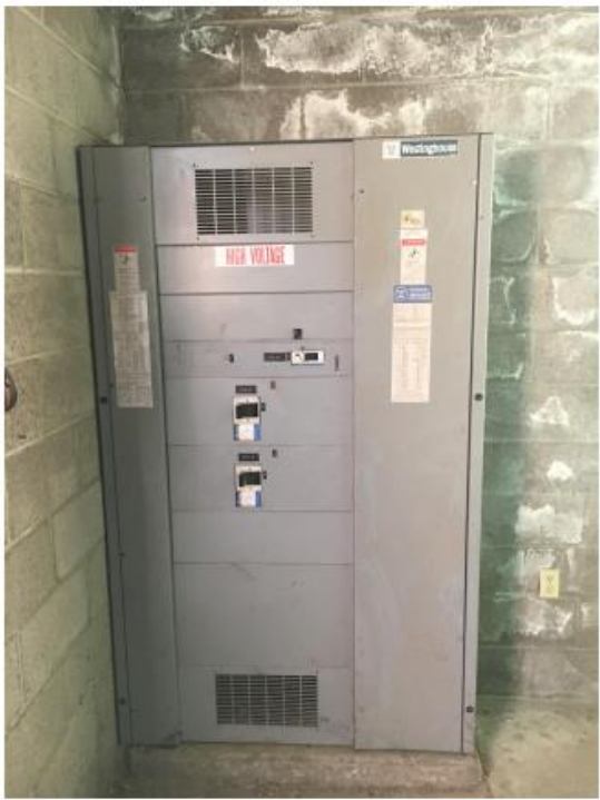
2 - Generator distribution panel not indicated on single line diagrams. 1200A, 277/480V, 3-phase, 4-wire.
