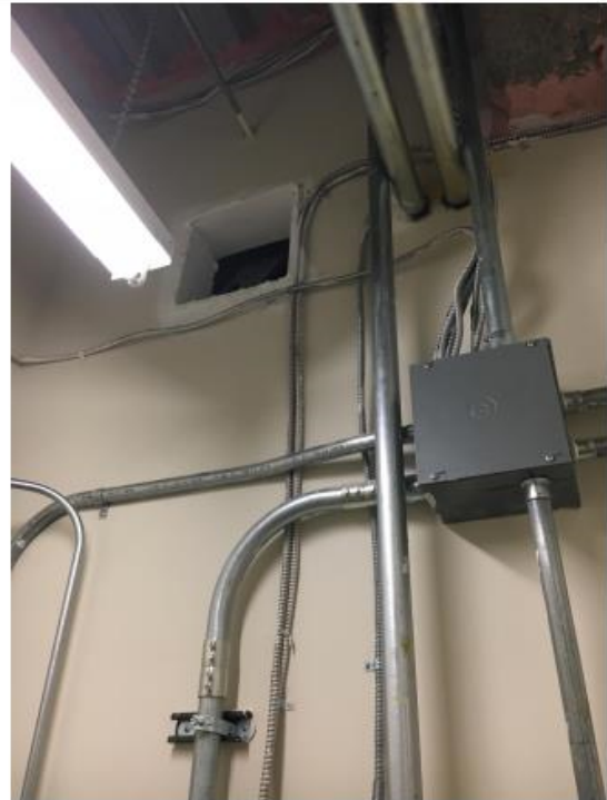
4 - Hole observed in rated wall of emergency electrical room on level 2.
