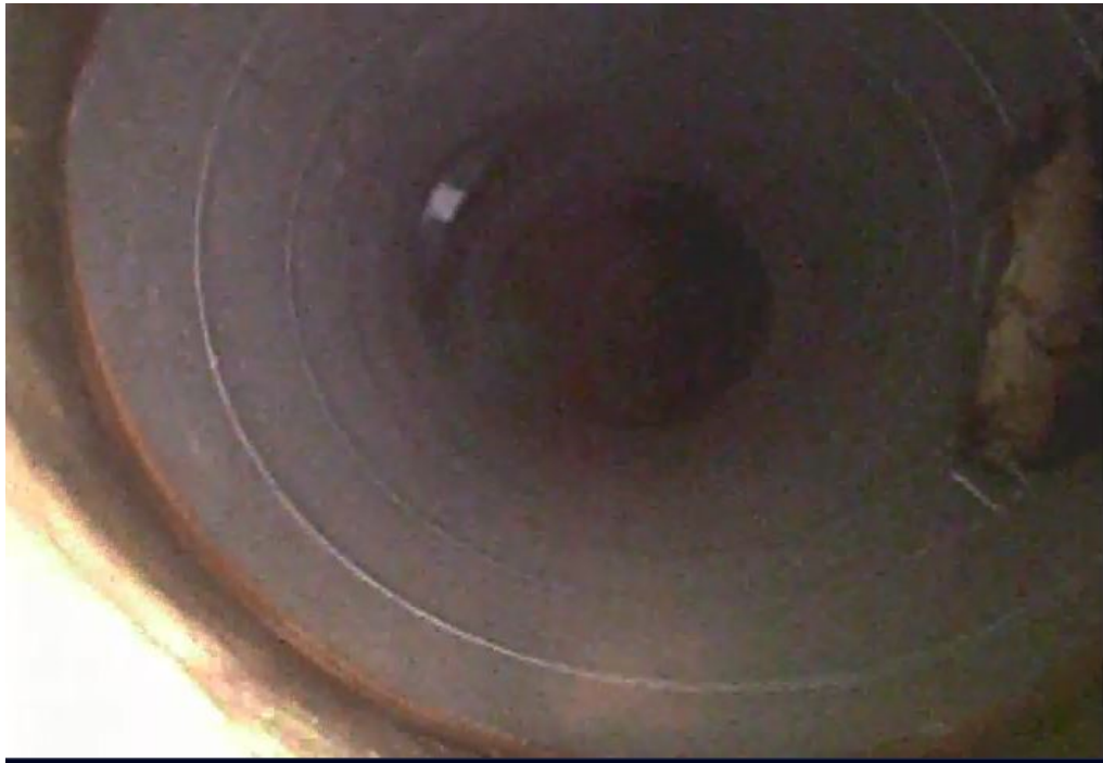
2 - Duct Sections - Branch Penetration - Exposed Insulation
