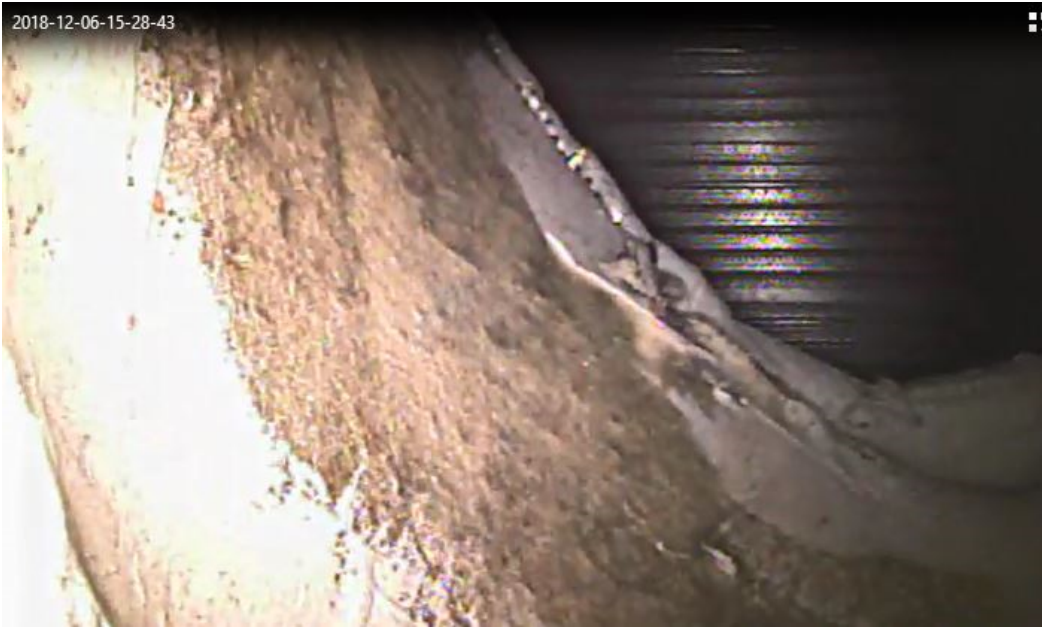
3 - Duct Reducing - Exposed Fiberglass and Poor Insulation
