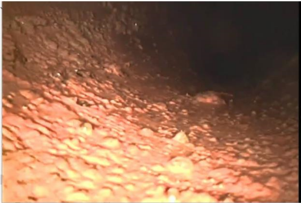
1 - Hydronic Piping - Interior Condition
