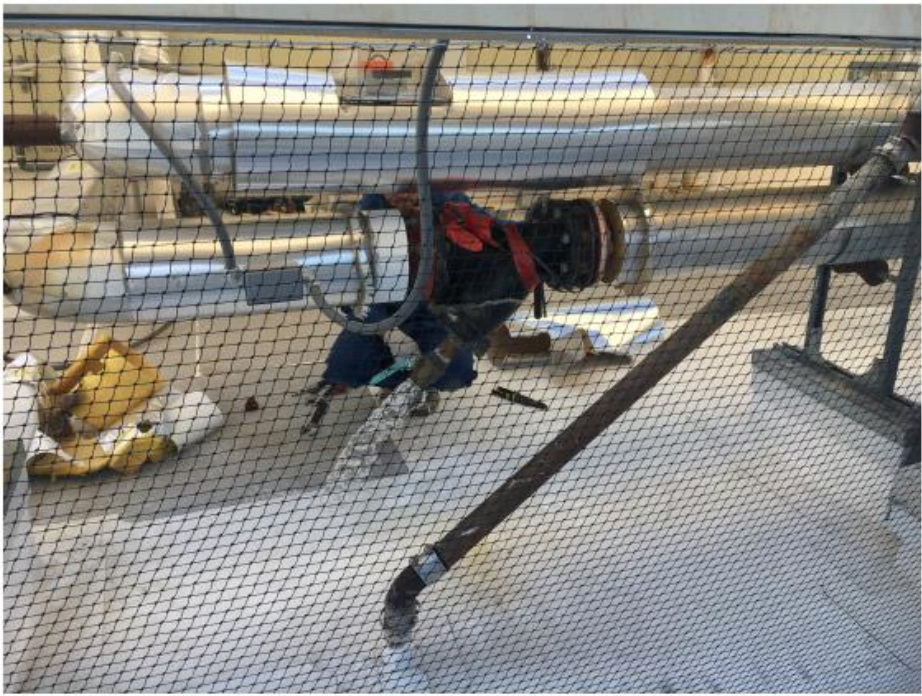
5 - Hydronic Piping - Camera Insertion Point
