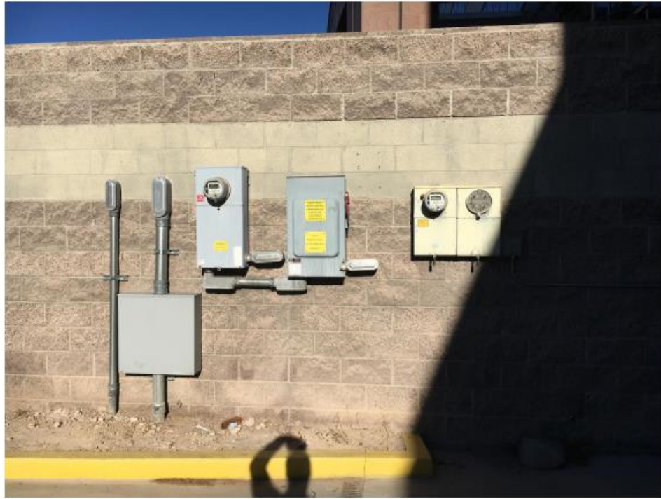
1 - Meters located at north end of building near loading dock. NVE meter is on the right. The PV system REC meter is on the left.
