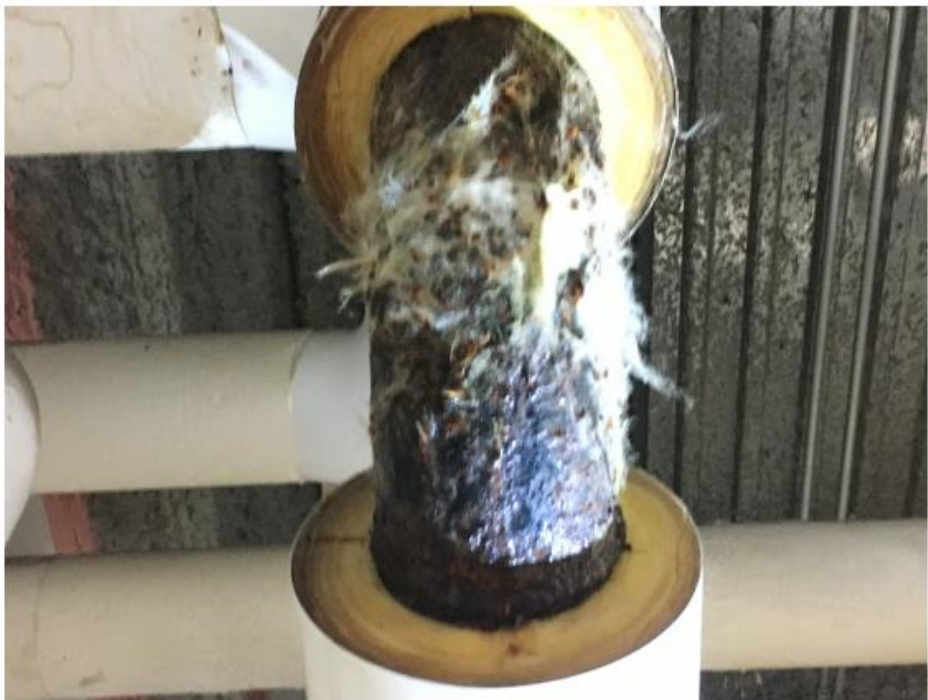
5 - Hydronic Piping - Exterior Corrosion & Insulation
