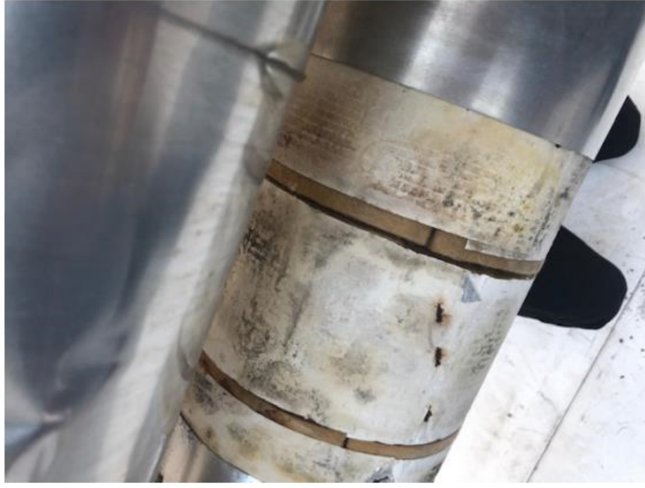
2 - Hydronic Piping - Exterior Insulation
