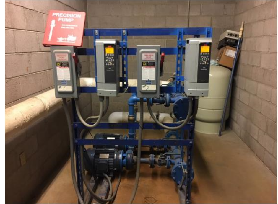
3 - Plumbing Systems - Domestic Booster Pump
