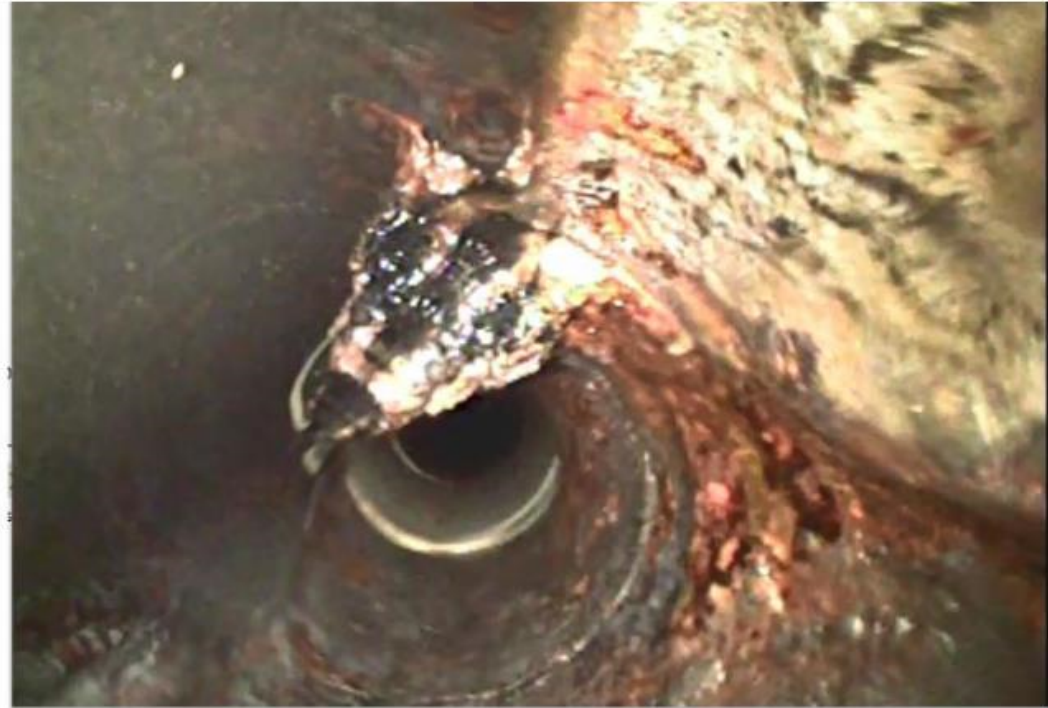
5 - Plumbing Systems - Collapsed Cast Iron
