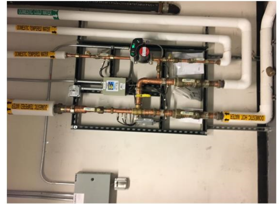
3 - Plumbing Systems - Tempering Station
