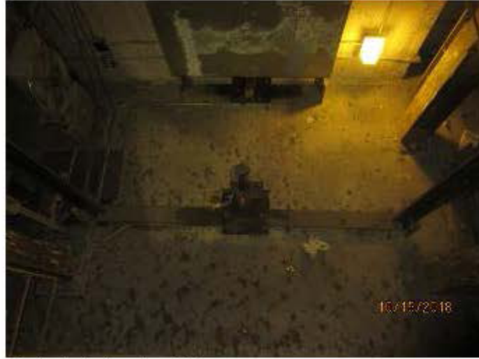
Typical pit showing buffer.
