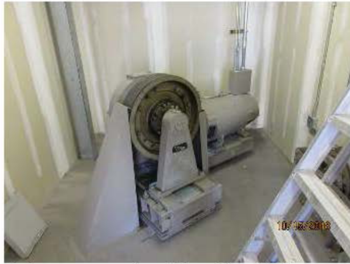
Service car worm and gear DC machine with DC motor.
