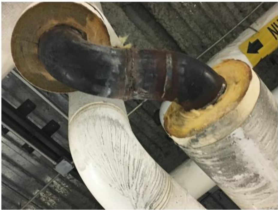
6 - Hydronic Piping - Exterior Condition & Insulation
