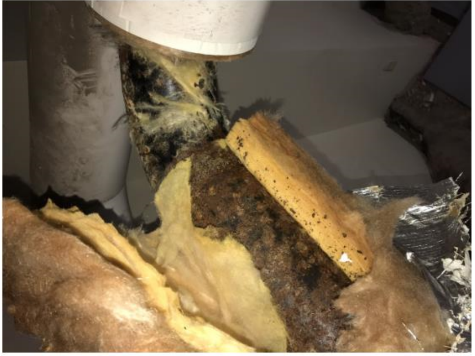
3 - Hydronic Piping - Exterior Corrosion & Insulation
