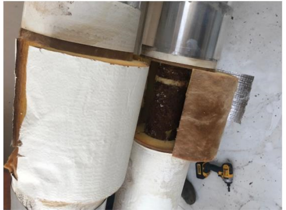
6 - Hydronic Piping - Exterior Condition & Insulation
