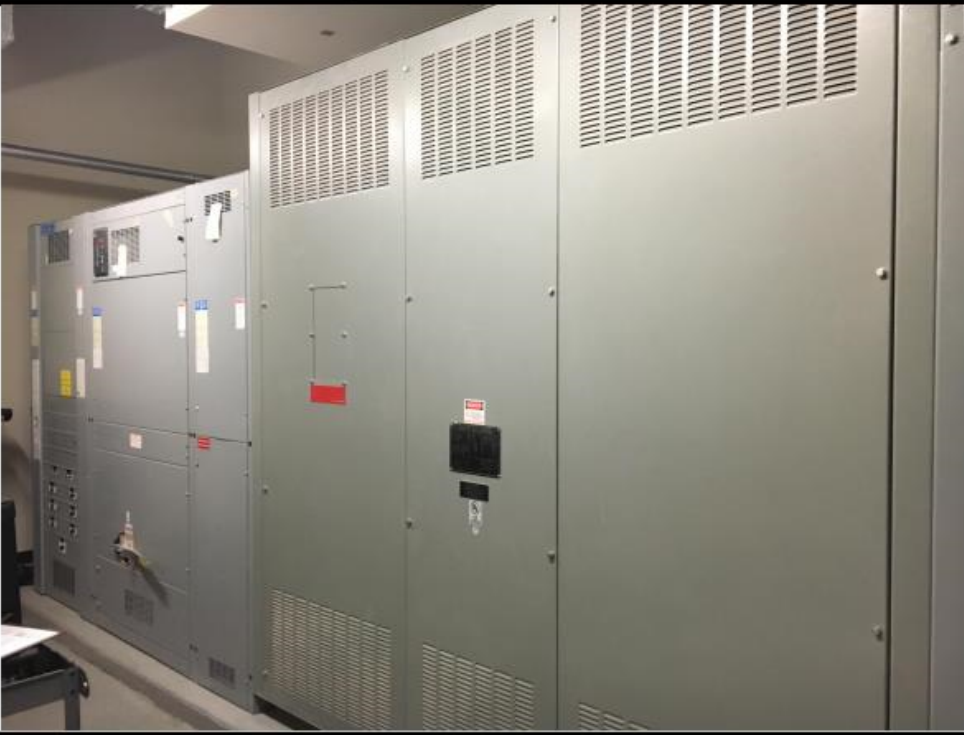
4 - Unit-substation 'USW' located on west half of Level 1. (1500kVA) Equipment is mis-labeled as 'USR'.
