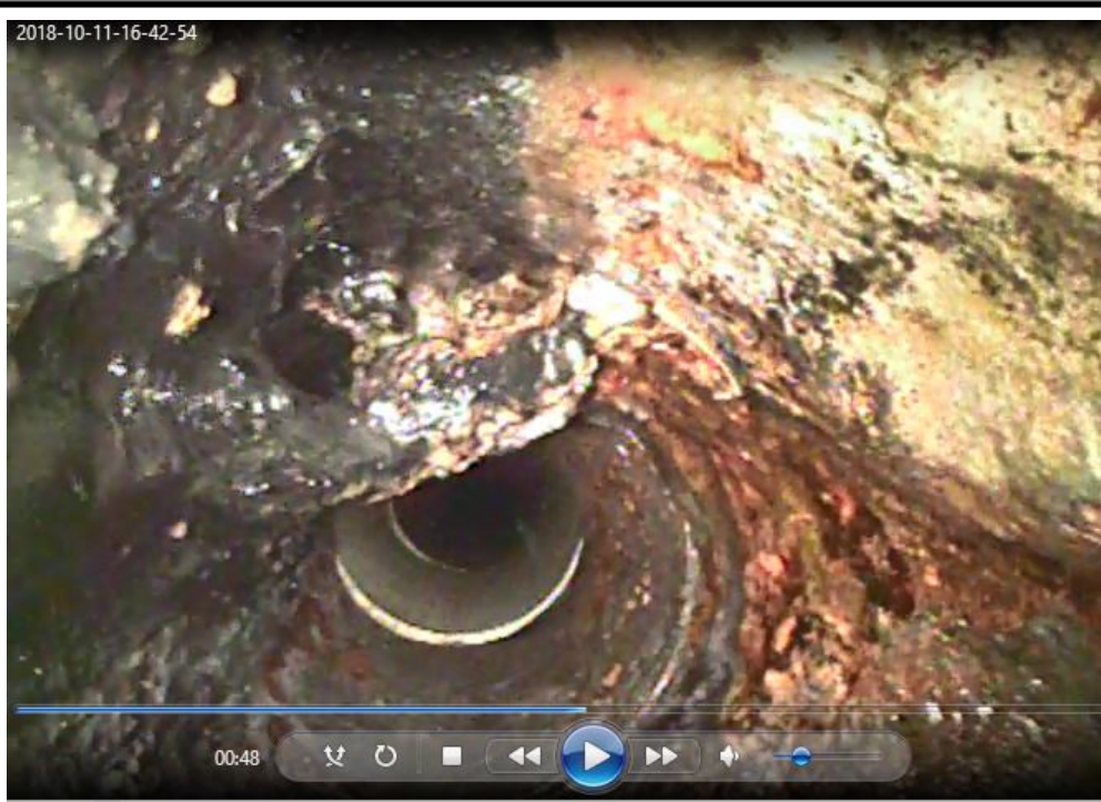
3 - Plumbing Systems - Underground - Collapsed Cast Iron
