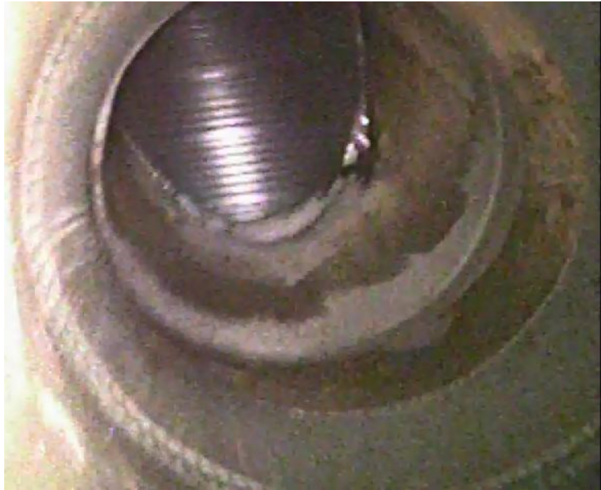
1 - Duct Reducing Fitting with Mastic Sealant
