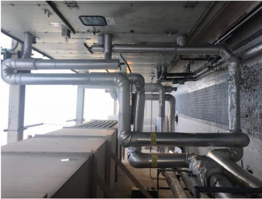
5 - Hydronic Piping - AHU Connection
