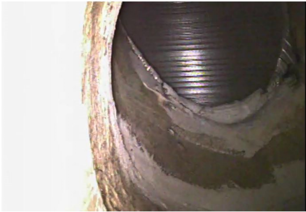
2 - Duct Reducing Fitting with Mastic Sealant
