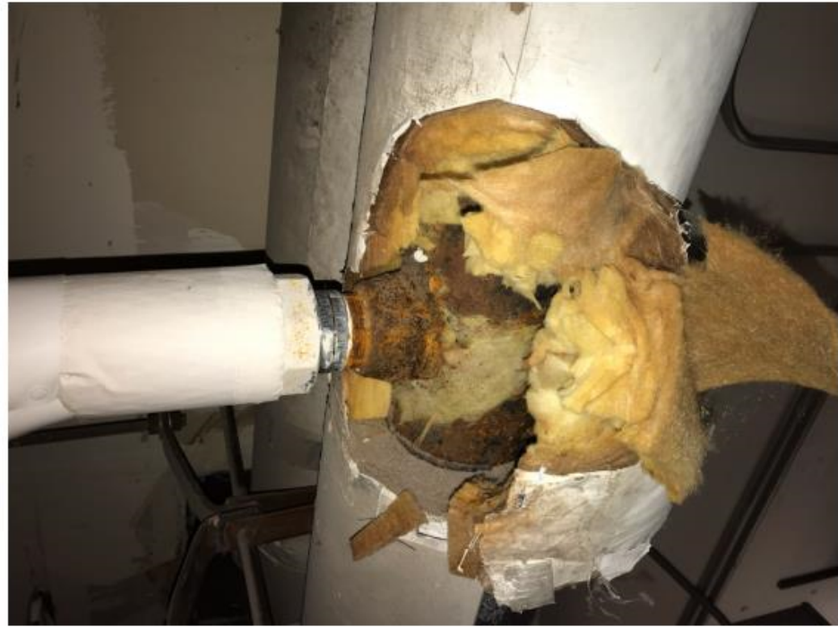
4 - Hydronic Piping - Exterior Corrosion & Insulation
