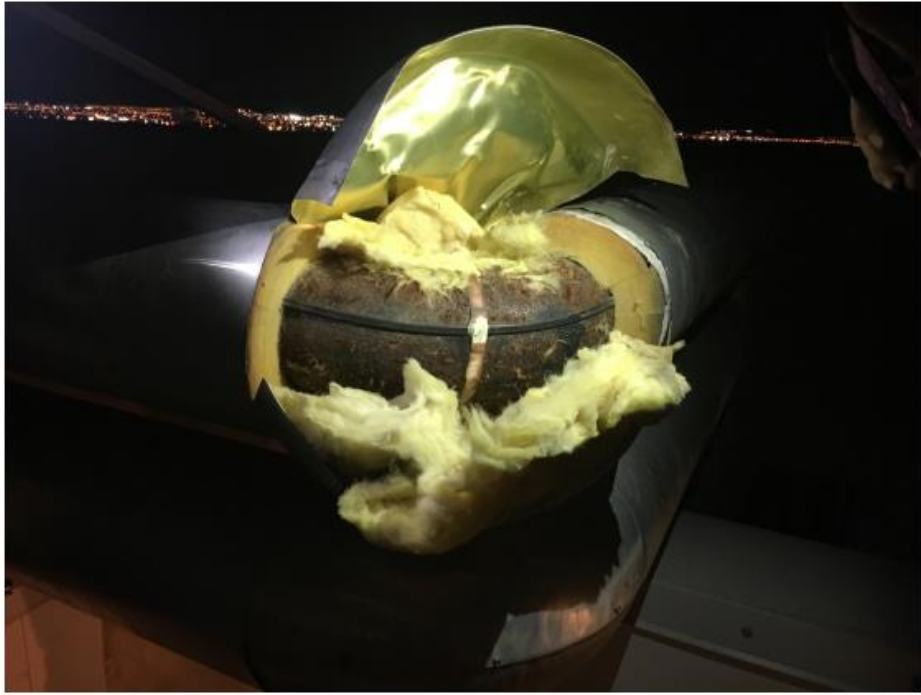
1 - Hydronic Piping - Exterior Corrosion & Insulation
