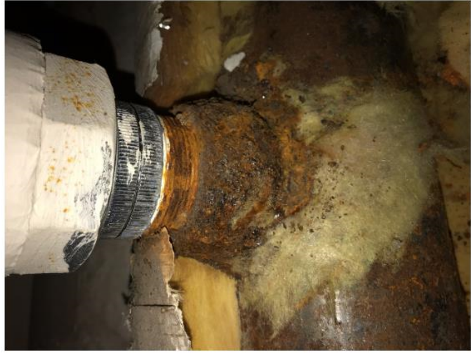
5 - Hydronic Piping - Exterior Corrosion & Insulation
