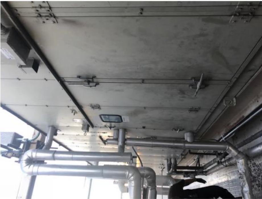
4 - Hydronic Piping - AHU Connection
