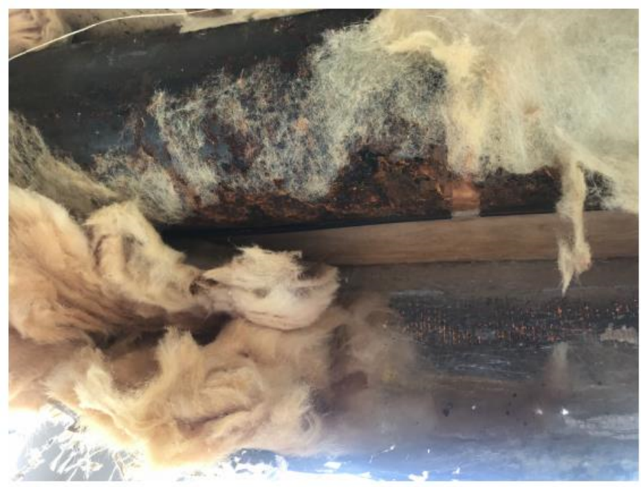
1 - Hydronic Piping - Exterior Corrosion & Insulation
