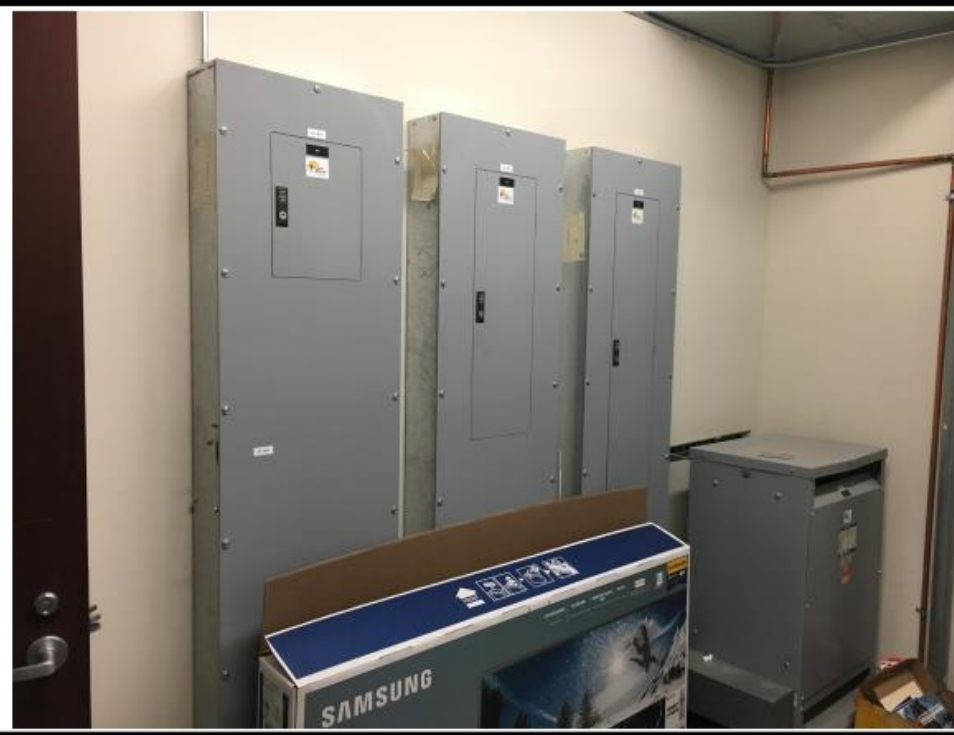
5 - Electrical room on west half of Level 1 adjacent to Cafe. Electrical rooms should not be used for storage.
