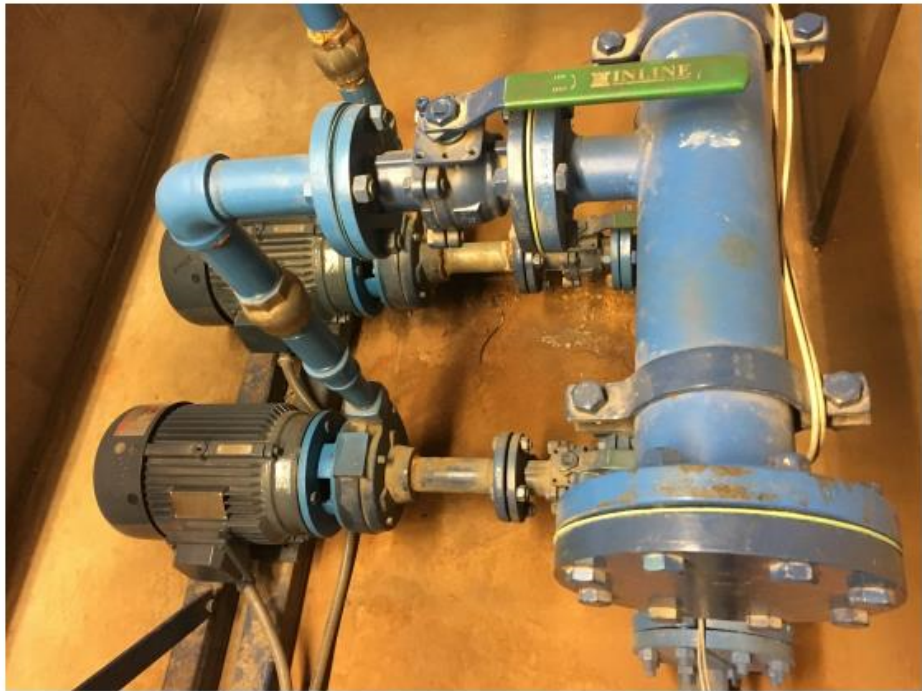
1 - Plumbing Systems - Domestic Booster Pump
