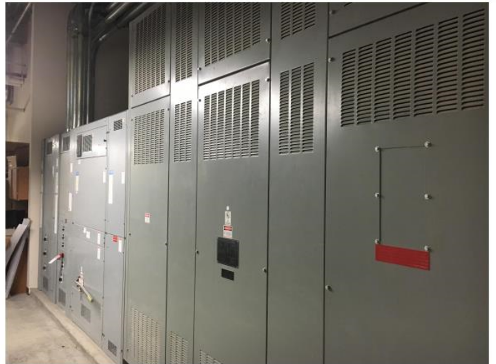
6 - Unit-substation 'USR' located on Level 6. (2500kVA) Equipment is mis-labeled as 'USW'.
