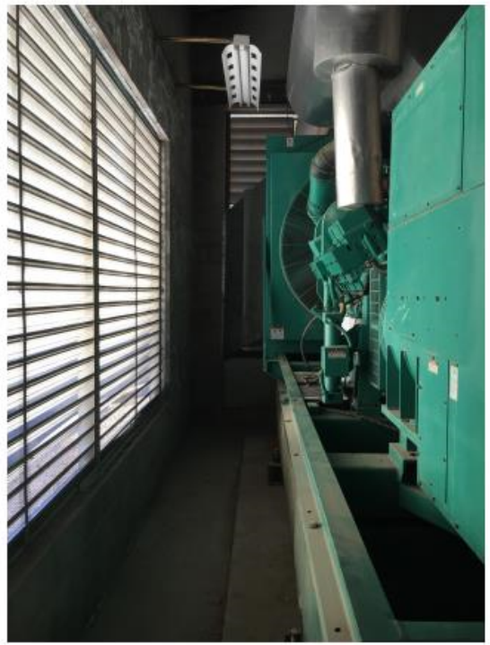
1 - Generator. 800kW, 277/480V, 3-phase, 4-wire with 500 gallon sub-base fuel tank.
