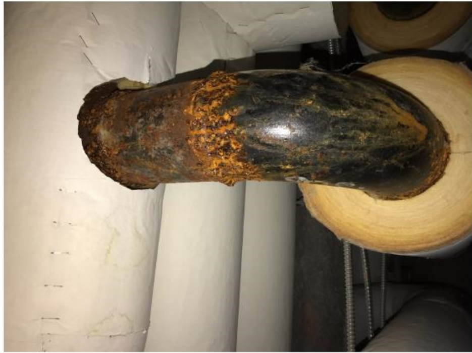
1 - Hydronic Piping - Exterior Condition & Insulation
