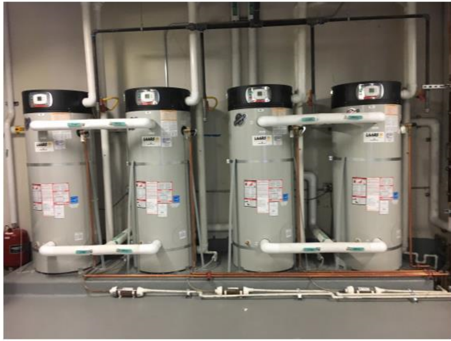
1 - Plumbing Systems - Water Heaters
