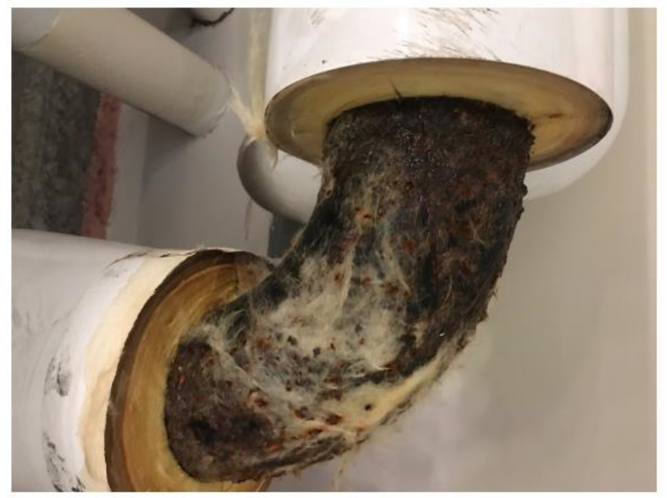
3 - Hydronic Piping - Exterior Corrosion & Insulation
