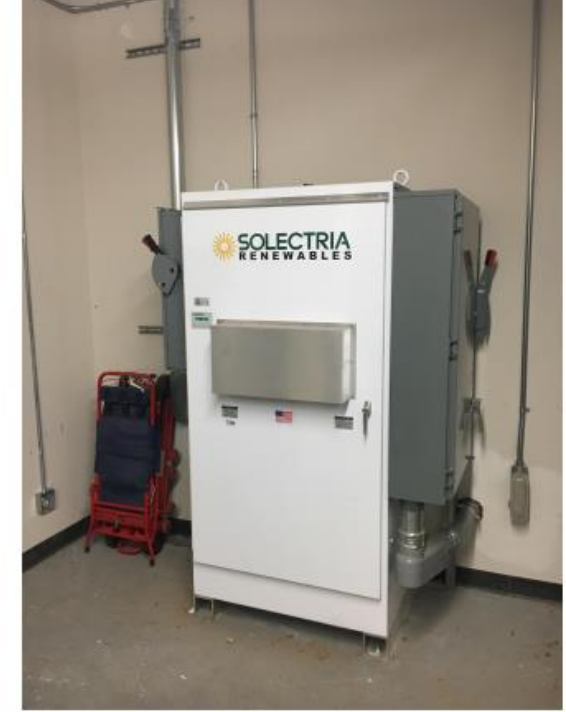
3 - PV system inverter located in same room as main service switchgear. Inverter is tied into service at 480V Unit-substation 'USW'.
