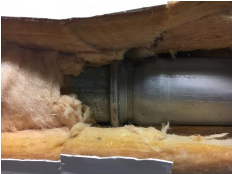
3 - Hydronic Piping - Heating Hot Water
