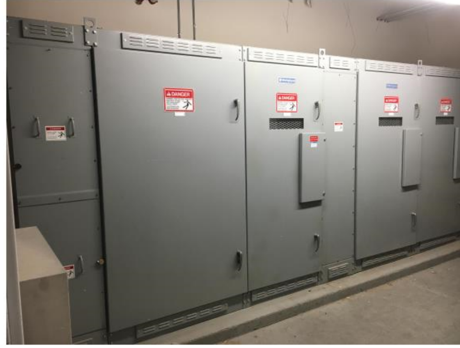
2 - Main service switchgear 'MVS1' 600A, 12.47KV, 3-phase, 3-wire.
