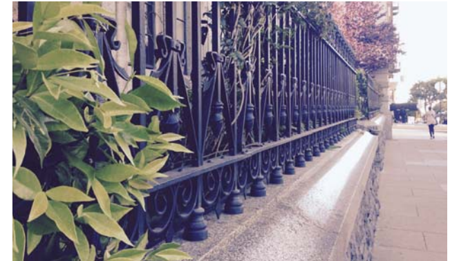
Decorative iron fence set on elevated stone wall, collars at base hide attachment sleeves, Nob Hill, San Francisco, CA, photo by M. Schmitter April 2015.
