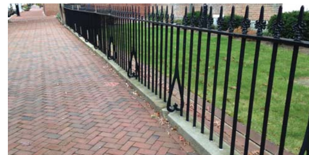
Wrought iron fence set on a granite base with lead sleeves, circa 1840, Lancaster, PA, photo by M. Schmitter, November 2014.
