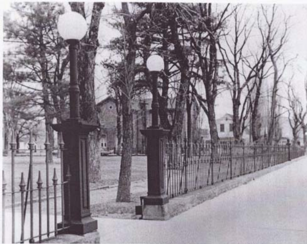
Circa 1950 photograph of Capitol Fence at secondary axis with 1911 light extensions to cast end posts apparent, backstays in original locations, Nevada State Museum #CM-5327-P-00057.
