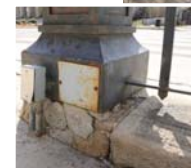
Note footing and electrical repairs on 1980 light fixture addition.
