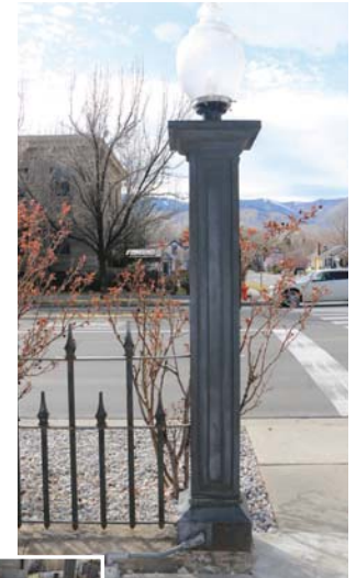
Note footing and electrical repairs on 1980 light fixture addition.
