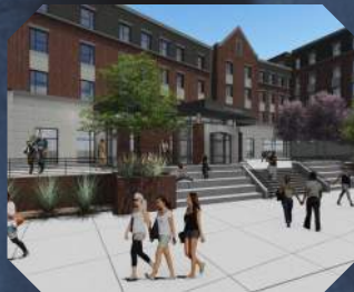
University of Nevada, Reno Great Basin Hall
