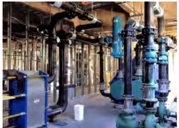
Above: BIM solutions at work in the mechanical-chiller room. The team used clash detection to improve field efficiency and avoid costly revisions.
